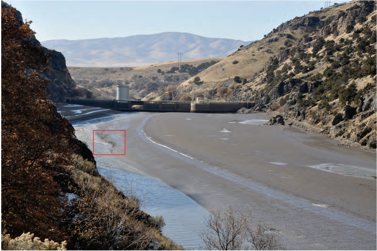
Photo 1. Looking downstream (westerly) towards Cutler Dam from the south side of Cutler Canyon during the 2019 full drawdown (November 4). Water surface elevation (WSE) at Cutler Dam was 4,386.97 (NGVD29), approximately 17 feet below the lowest proposed operating level of 4,405.0. Note that the majority of the bank longitudinally and laterally is stable under this extreme drawdown event except for a limited area delineated by the red square.
