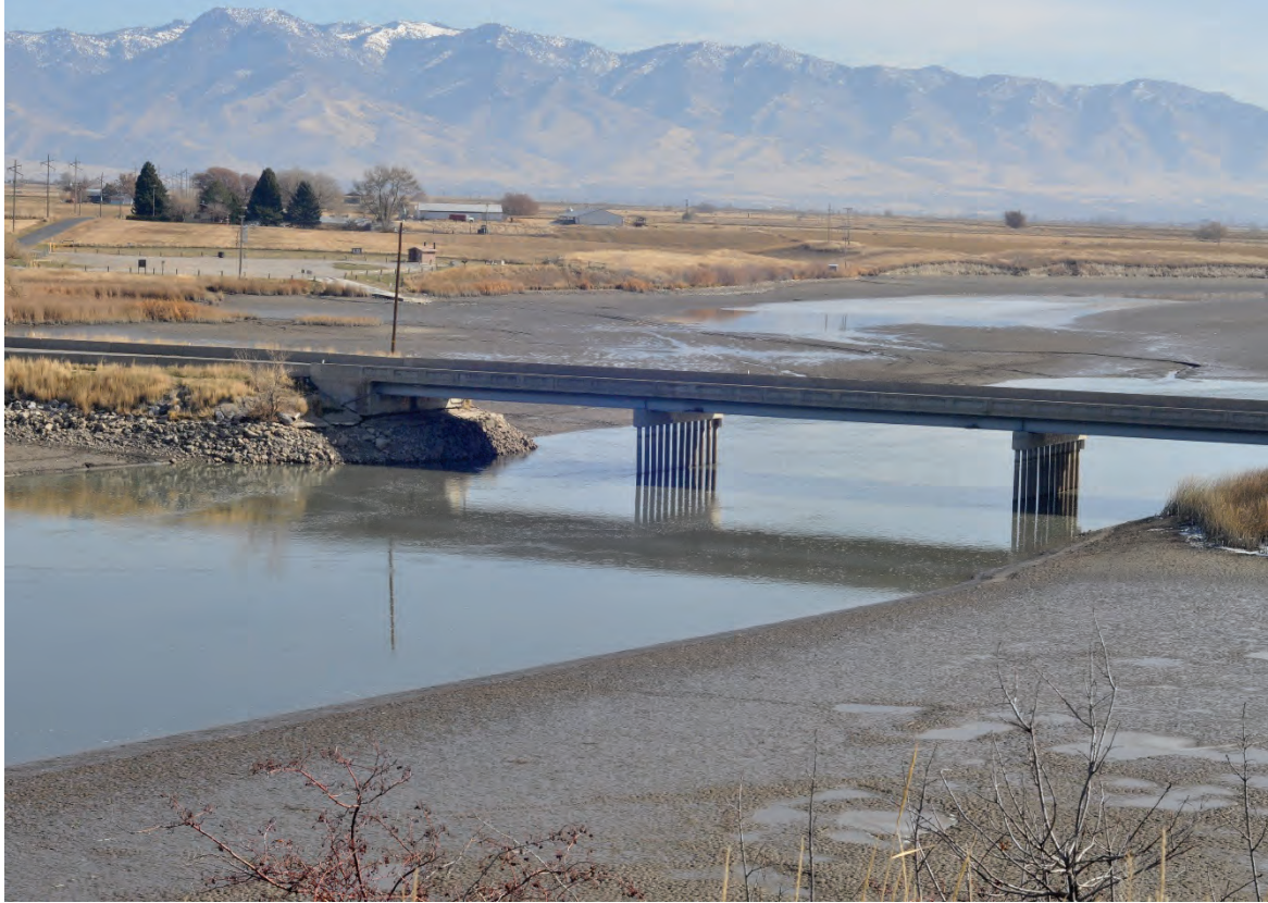
Photo 3. Downstream of Newton Bridge looking upstream toward easterly bank with PacifiCorp's Cutler Canyon Recreation Site in the background. Note the lack of head-cutting in the exposed reservoir bed and along the wetted perimeter. WSE in this reach is hydraulically controlled by Wheelon Dam during the 2019 extreme drawdown event, approximately 17 feet below the lowest proposed operating limit. Photo taken on November 4, 2019, same WSE as Photos 1 and 2.
