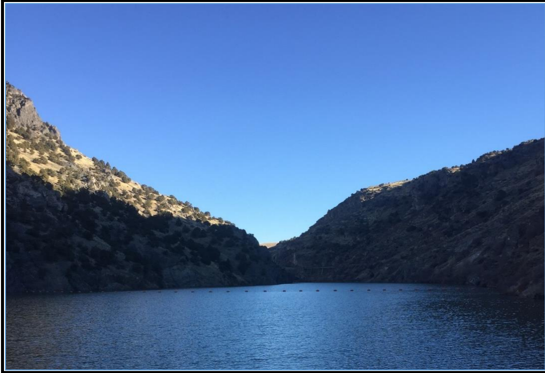
PHOTO 2-1 CUTLER RESERVOIR LOOKING UPSTREAM (EAST) FROM CUTLER DAM
