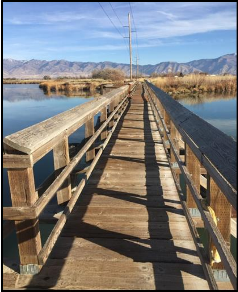
PHOTO 3-8 BENSON RAILROAD BRIDGE TRAIL AND FISHING BRIDGE
