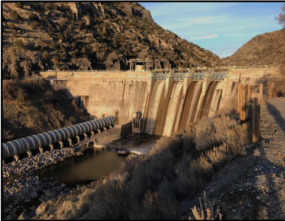
PHOTO 3-11 DOWNSTREAM FACE OF CUTLER DAM, LOOKING NORTHEAST INTO CUTLER CANYON
