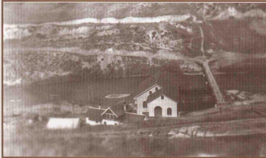
Third addition - When the Wheelon Plant was increased to 5400 horse power in 1906. Note the supply pipe has a plant deck. It was also used as a bridge.
