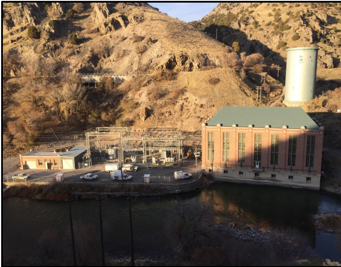
PHOTO 2-7 POWERHOUSE, SURGE TANK, AND (NON-PROJECT) SUBSTATION
