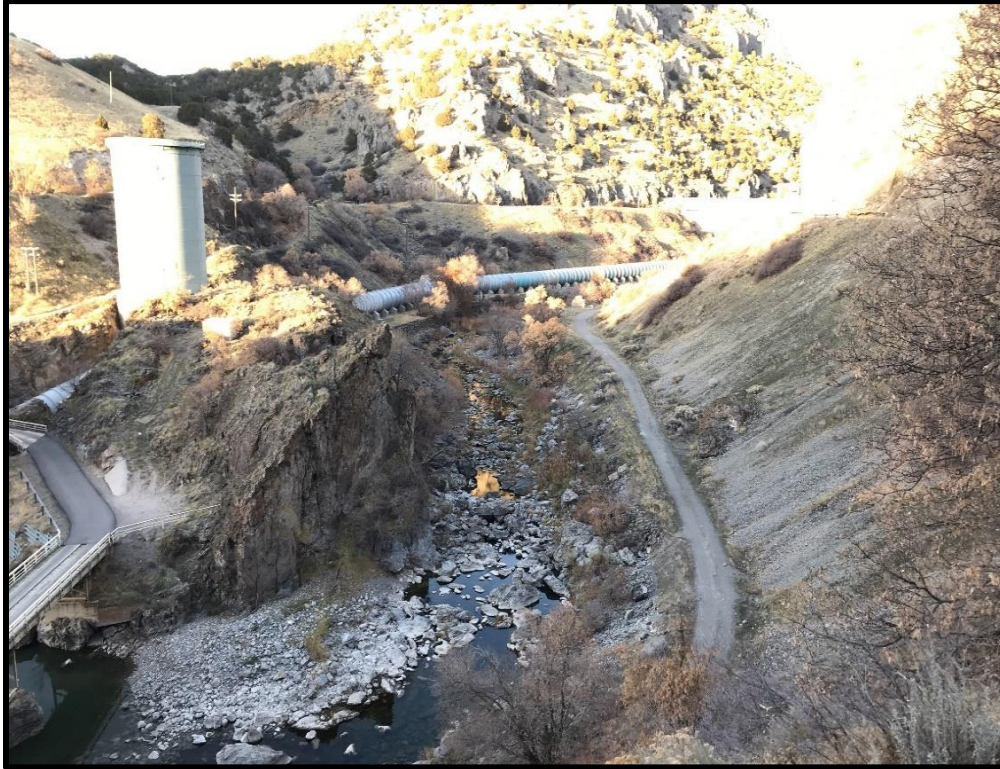
PHOTO 3-12 FLOWLINE AND SURGE TANK, LOOKING UPSTREAM FROM THE POWERHOUSE AT THE BYPASSED REACH
