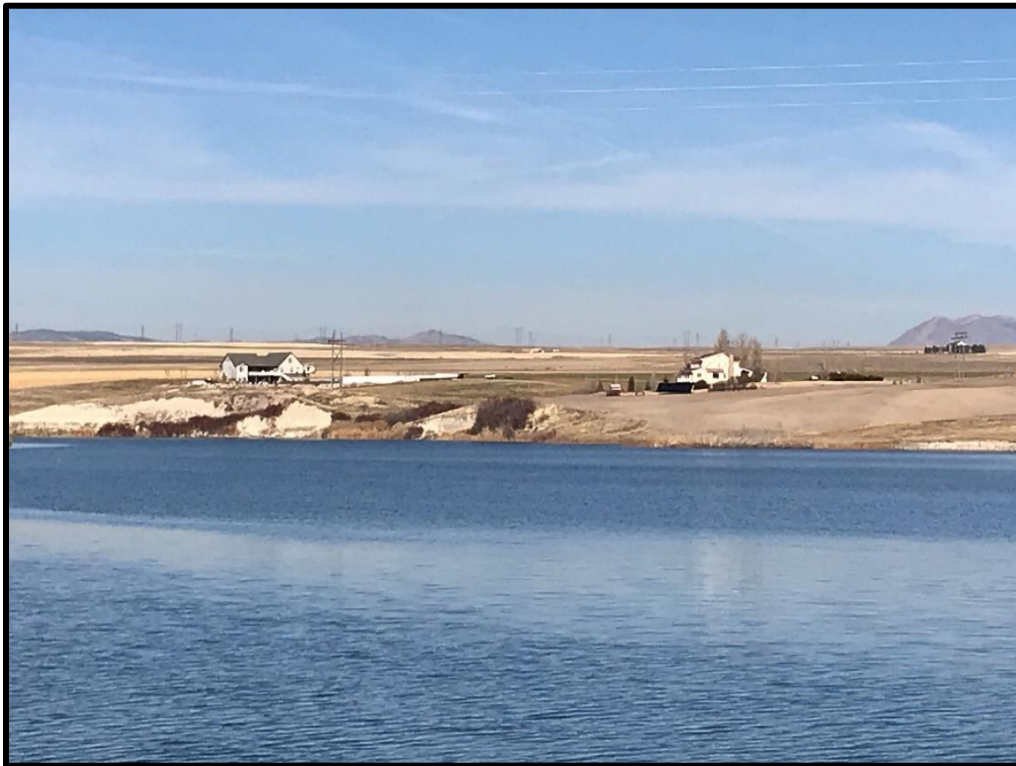
PHOTO 3-17 CUTLER RESERVOIR NEAR NEWTON, UTAH IN THE CUTLER CANYON MANAGEMENT UNIT
