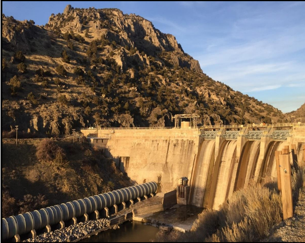
PHOTO 2-2 CUTLER DAM, PENSTOCK, AND SPILL GATES FROM DOWNSTREAM
