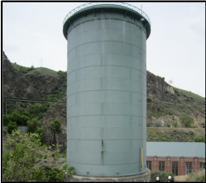
PHOTO 2-6 CUTLER JOHNSON DIFFERENTIAL SURGE TANK
