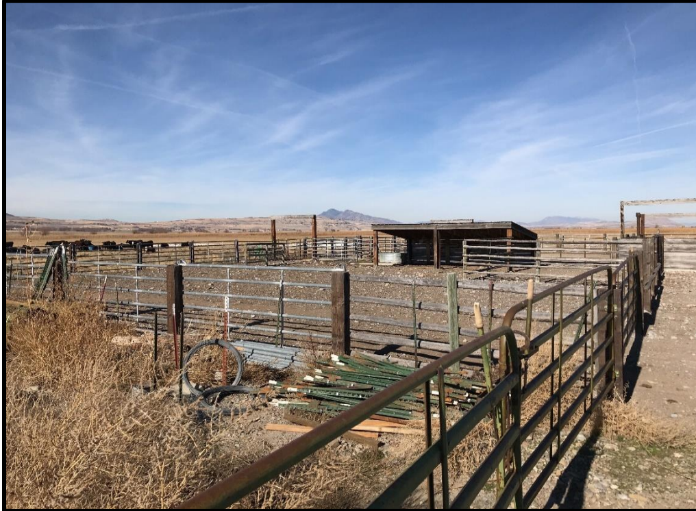
PHOTO 3-26 CATTLE FENCING AND CORRAL STRUCTURES IN THE SOUTH MARSH MANAGEMENT UNIT
