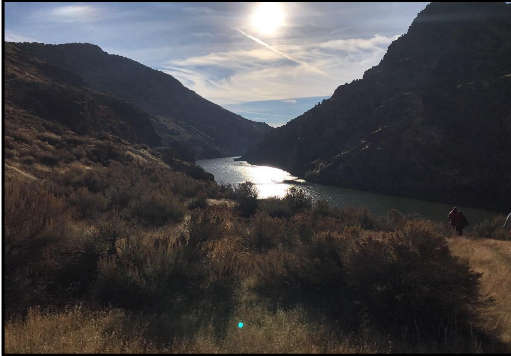
PHOTO 3-14 CUTLER RESERVOIR IN CUTLER CANYON MANAGEMENT UNIT, LOOKING DOWNSTREAM NEAR HISTORIC WHEELON DAM LOCATION
