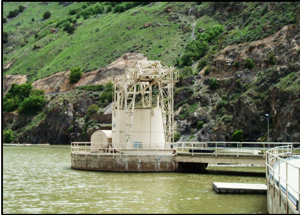
PHOTO 2-4 CUTLER FLOWLINE INTAKE STRUCTURE
