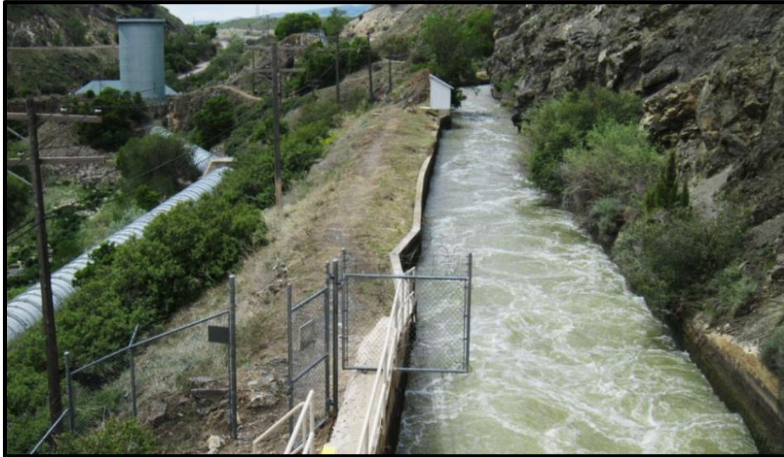
PHOTO 2-3 LOOKING DOWNSTREAM AT WESTSIDE CANAL
