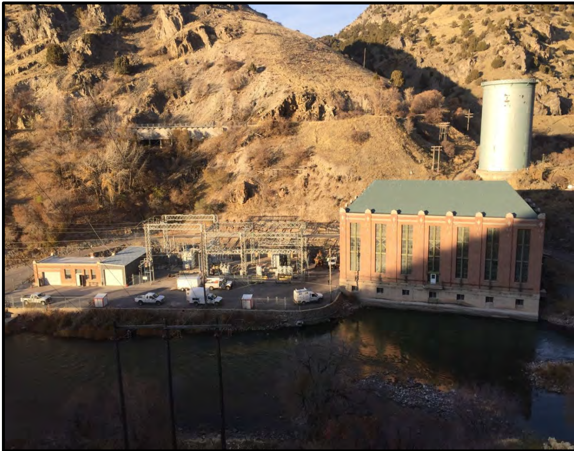
PHOTO 2-7 POWERHOUSE, SURGE TANK, AND (NON-PROJECT) SUBSTATION
