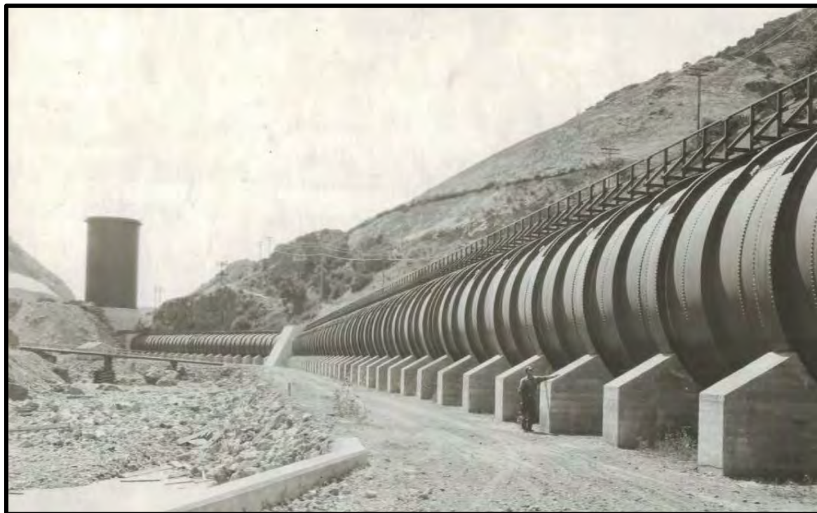
PHOTO 3-2 FLOWLINE CONSTRUCTION IN BEAR RIVER CANYON, UTAH, 1925-1927
