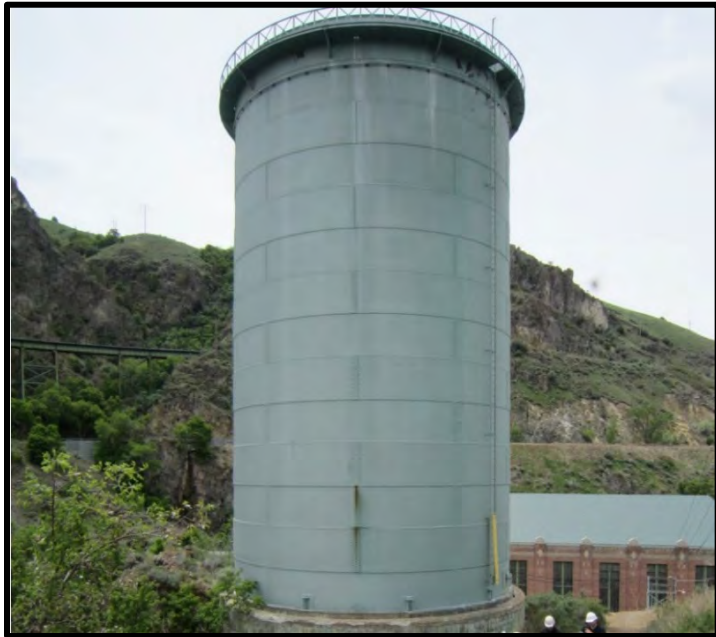
PHOTO 2-6 CUTLER JOHNSON DIFFERENTIAL SURGE TANK
