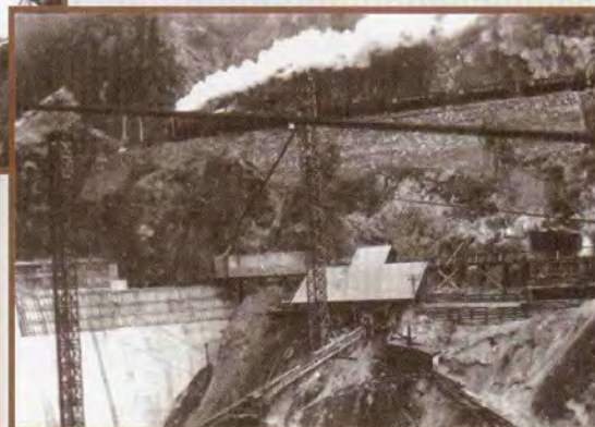
Two cement mixers are under the shed. Sand and gravel are brought in by rail and lowered through pipes to a landing below.
