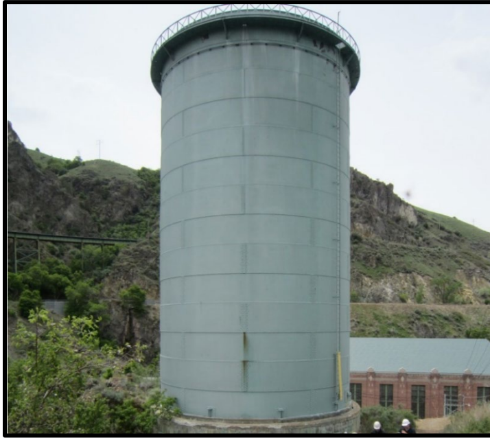
PHOTO 2-6 CUTLER JOHNSON DIFFERENTIAL SURGE TANK
