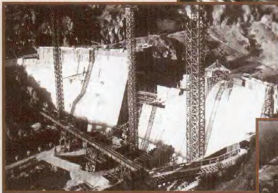
Lower side of dam conveyer is used to transport the cement to the hoists. Water is still being flumed beneath the dam.
