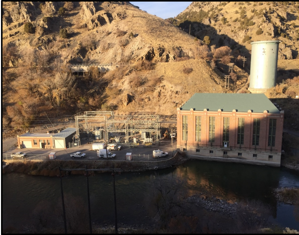
PHOTO 2-7 POWERHOUSE, SURGE TANK, AND (NON-PROJECT) SUBSTATION
