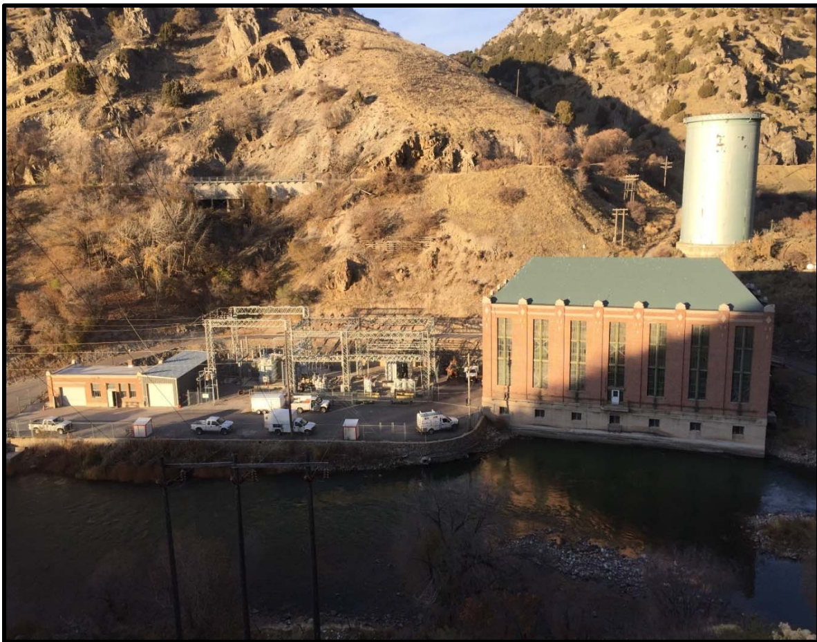
PHOTO 5-2 CUTLER HYDROELECTRIC POWERHOUSE, SURGE TANK AND SUBSTATION
