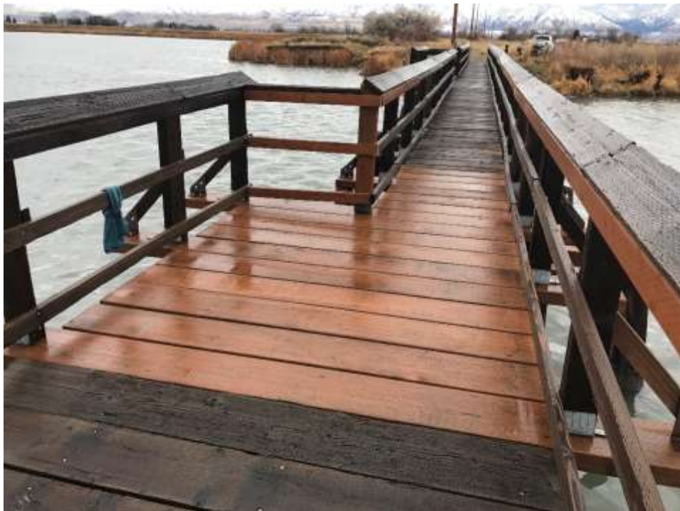
Photo D-4. Pedestrian Fishing Bridge Repair
