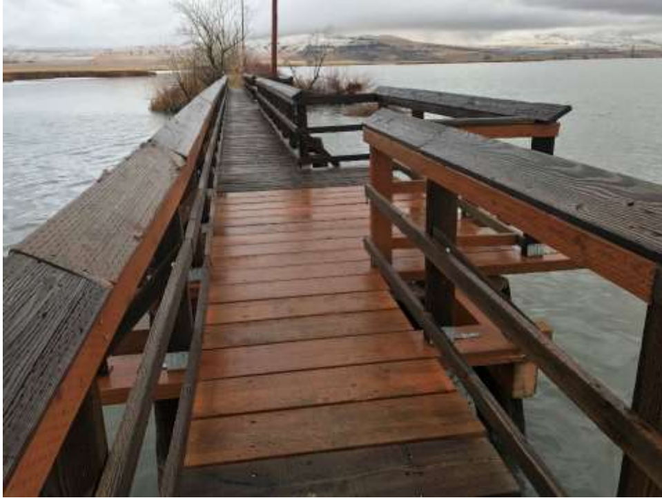
Photo D-3. Pedestrian Fishing Bridge Repair
