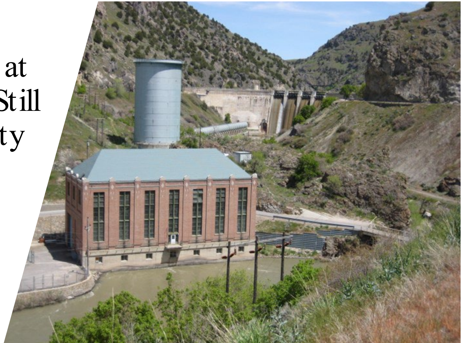
Cutler Powerhouse, Flowline, and Dam – Cutler Canyon walls in the background
