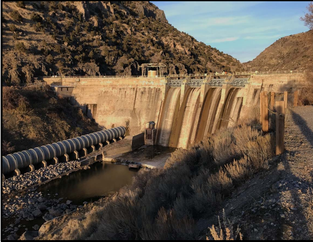
PHOTO 6-10 DOWNSTREAM FACE OF CUTLER DAM, LOOKING NORTHEAST
