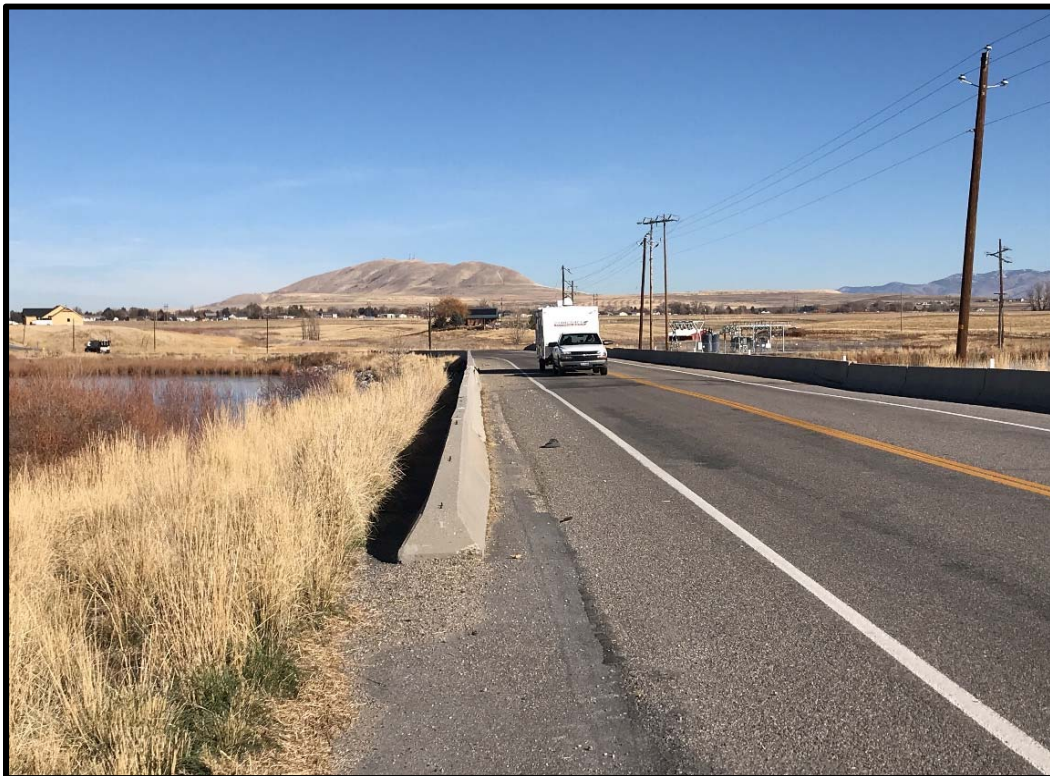
PHOTO 6-23 HIGHWAY 23 BRIDGE OVER CUTLER RESERVOIR NEAR NEWTON, UTAH, LOOKING NORTHEAST
