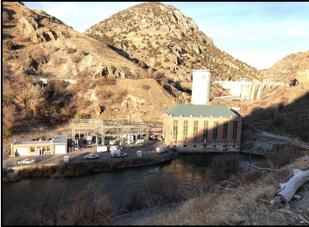
PHOTO 6-12 CUTLER POWERHOUSE AND SUBSTATION (NOT A PROJECT FEATURE), LOOKING UPSTREAM, CUTLER DAM IN THE BACKGROUND
