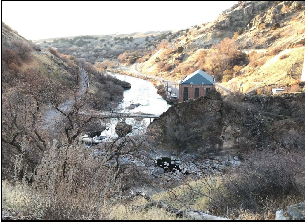
PHOTO 6-8 CUTLER POWERHOUSE WITH THE BYPASSED REACH IN THE FOREGROUND, LOOKING WEST FROM CUTLER CANYON
