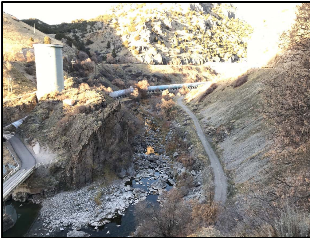
PHOTO 6-11 FLOWLINE AND SURGE TANK, LOOKING UPSTREAM FROM THE POWERHOUSE AT THE BYPASSED REACH
