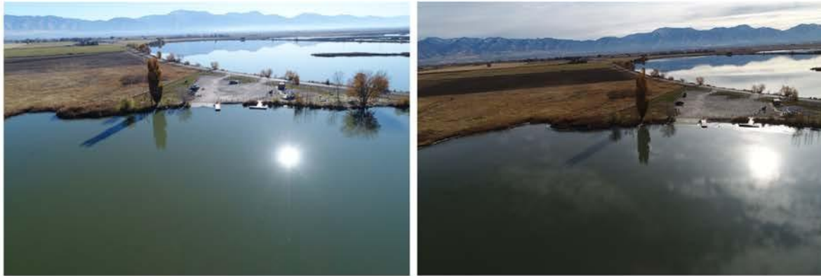
October 25, 2019, Cutler Dam elevation 4,407.22 October 28, 2019, Cutler Dam elevation 4,404.58
