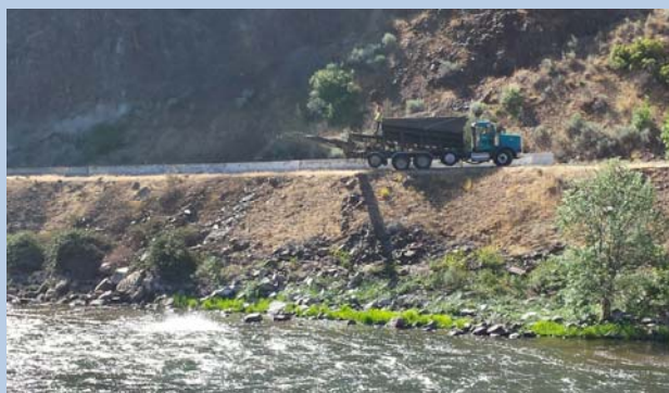
Gravel Augmentation Downstream of Iron Gate
