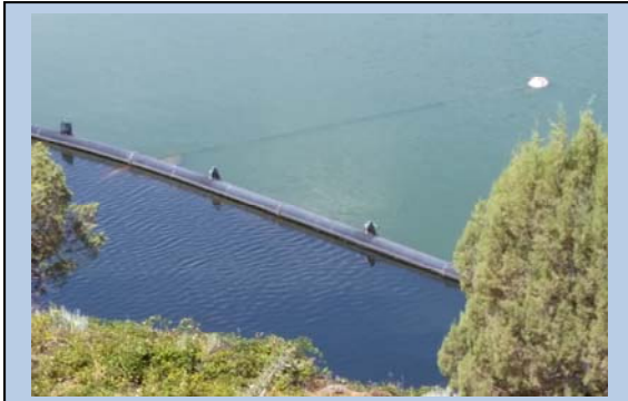
Iron Gate Reservoir on July 26, 2017 Showing Algae Upstream of Curtain and Clearer Water Downstream
