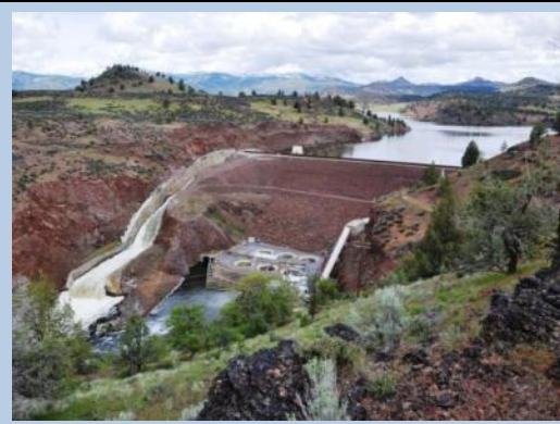
Iron Gate Dam and Powerhouse
