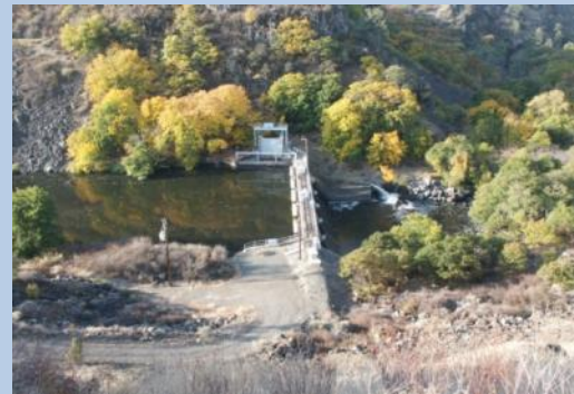
Copco No. 2 Dam
