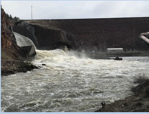
Approximately 9,500 cfs of Flow at Iron Gate Dam on April 10, 2019 at 8:30 AM (Photo: PacifiCorp)
