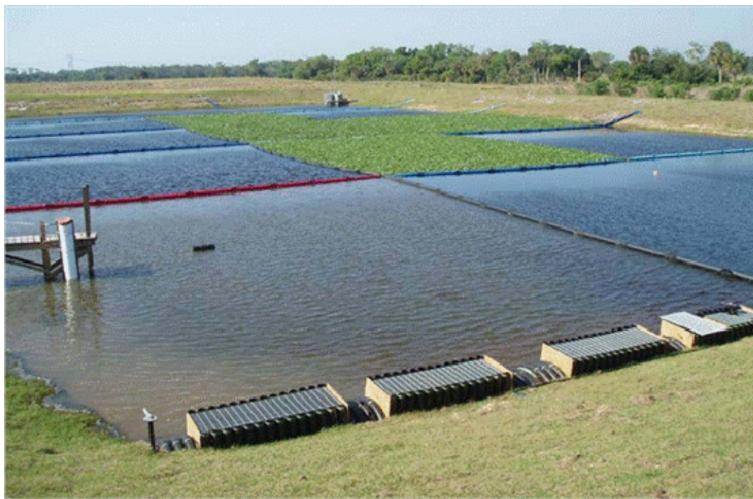
FIGURE 22 Hybrid Wetland Treatment Technology (HWTT) facility at Nubbin Slough in Florida (source: South Florida Water Management District).
