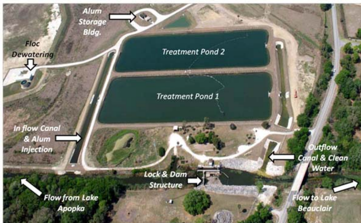
FIGURE 23 Aerial photograph of the Nutrient Reduction Facility (NuRF) in Florida (source: Lake County Water Authority).
