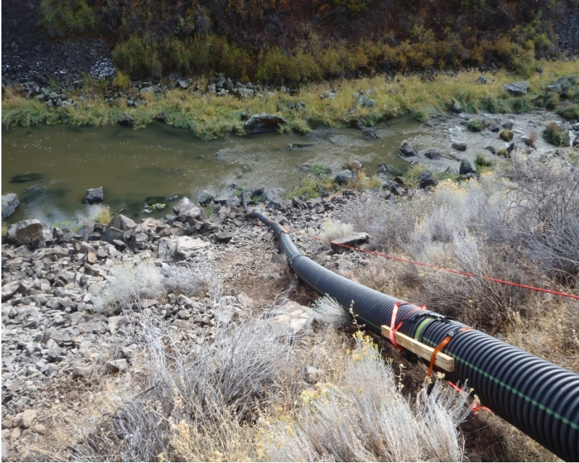
Figure 3.2-1. Gravel placement at RM 223.8 using a pipe.
