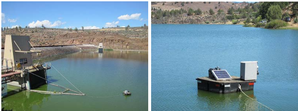
Figure 6. The vertical buoy device (B.O.B) is deployed upstream of the intake tower in Iron Gate Reservoir (August 2013).
