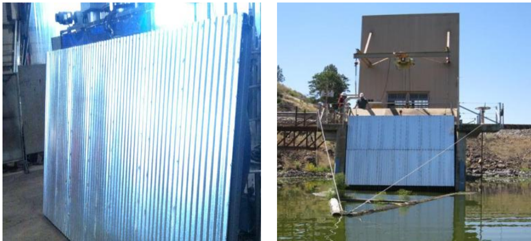
Figure 2. One of Two Steel Frames Shown Prior to Installation (left) and After Installation onto the Intake Tower (right).
