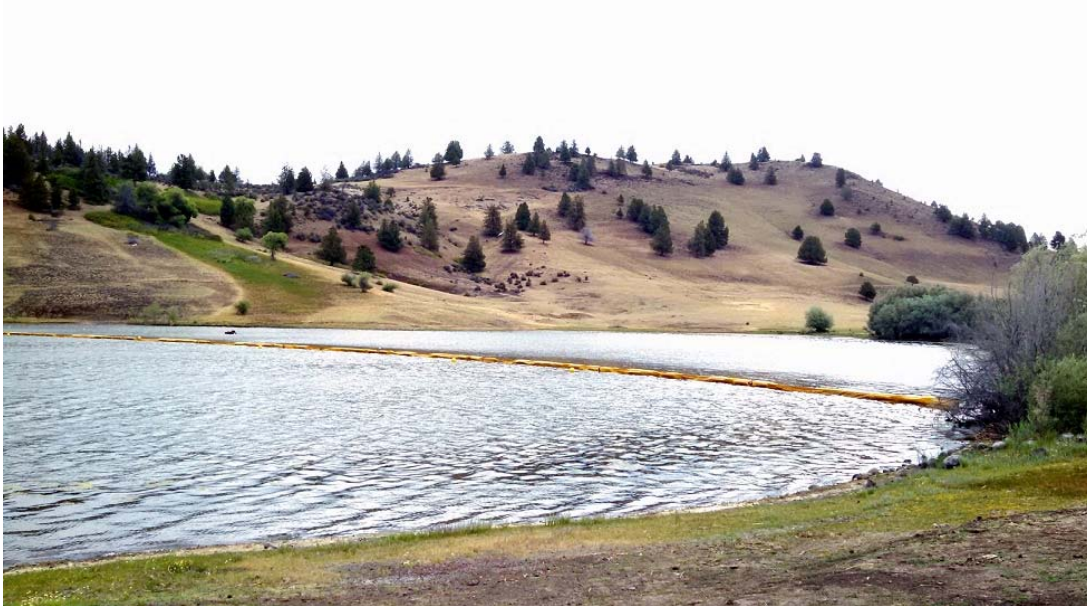
Figure 2. Curtain installed to isolate a portion of Long Gulch Cove.
