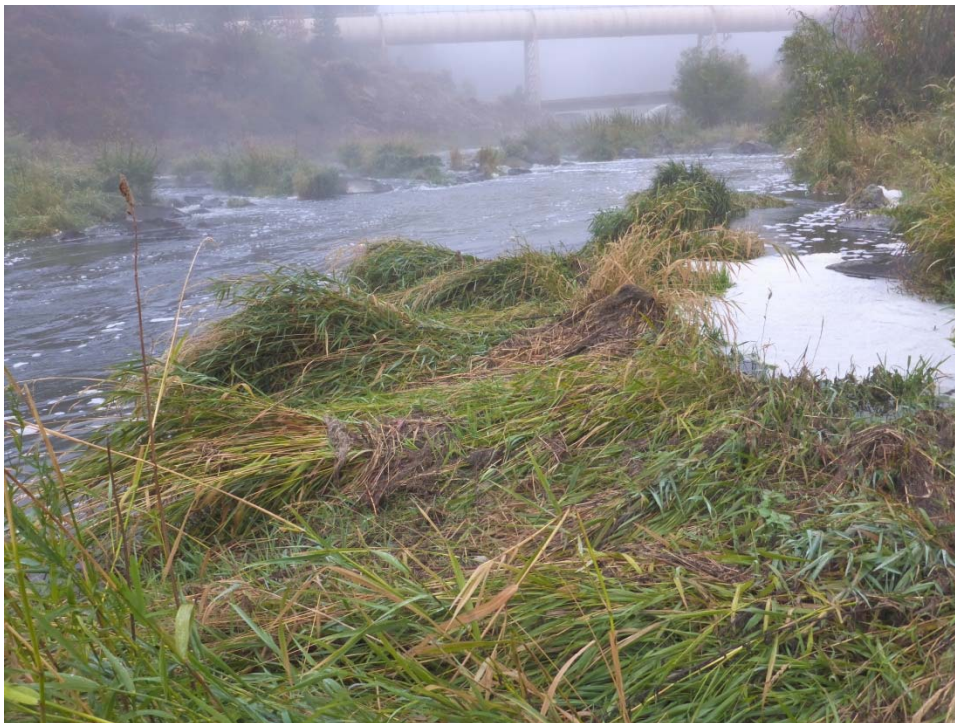
Figure 3.4-1. RM 224.5 Site showing evidence of flow over placed gravel bar (now vegetated).
