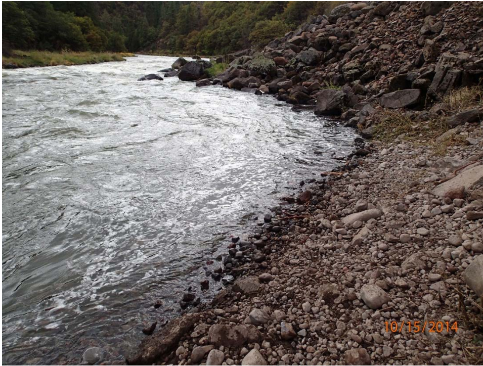
Figure 3.3-1. Photo of placed gravel at RM 219.9, October 2014 (just after placement).
