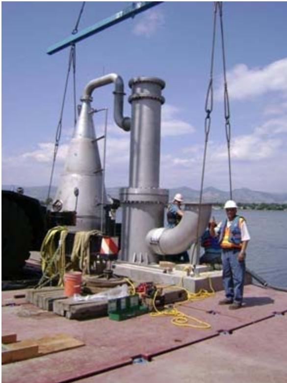
Figure 6. Example of a Speece cone installation readied for reservoir bottom placement. The Keno reservoir placement would be out of the water on the shore. Source: Image Eco2 Technologies.
