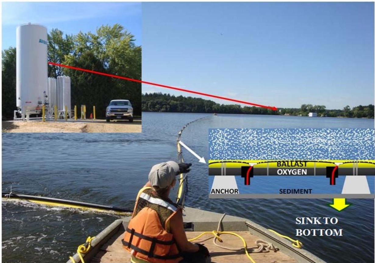
Figure 3. Example placement of linear diffuser for sparging of pure oxygen with diffuser. The diffuser system is manufactured at the water edge from HDPE pipe, floated on the surface close to shore during manufacture, and then sunk into position when completed. Oxygen supply in this instance is liquid oxygen. Source: CH2M unpublished project information with assistance from Mobley Engineering, Inc.
