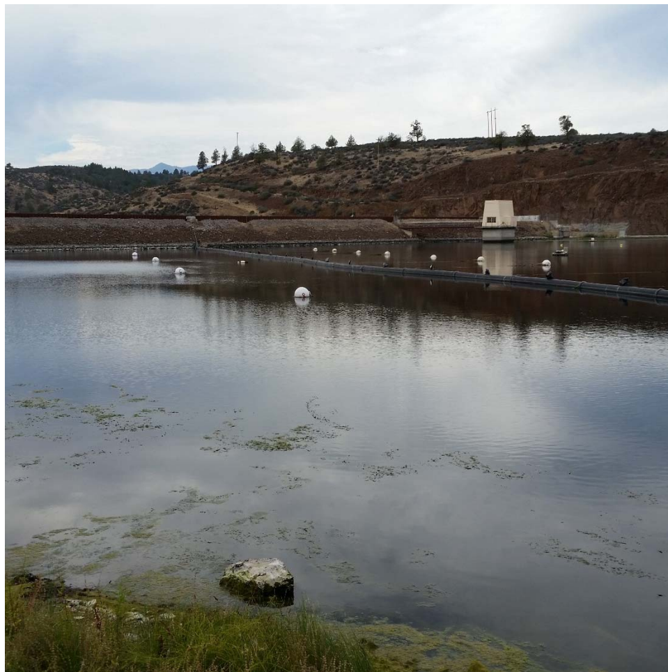
Figure 5-5. Photo of Iron Gate Reservoir (taken August 29, 2016) Showing Extensive Macrophyte Growth near the Shoreline.
