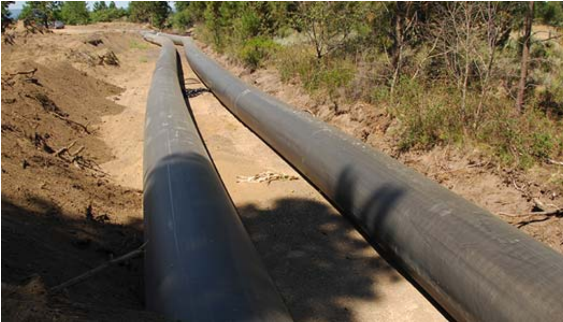
Figure 8. Irrigation efficiency and water management projects include water conveyance and piping improvements.
