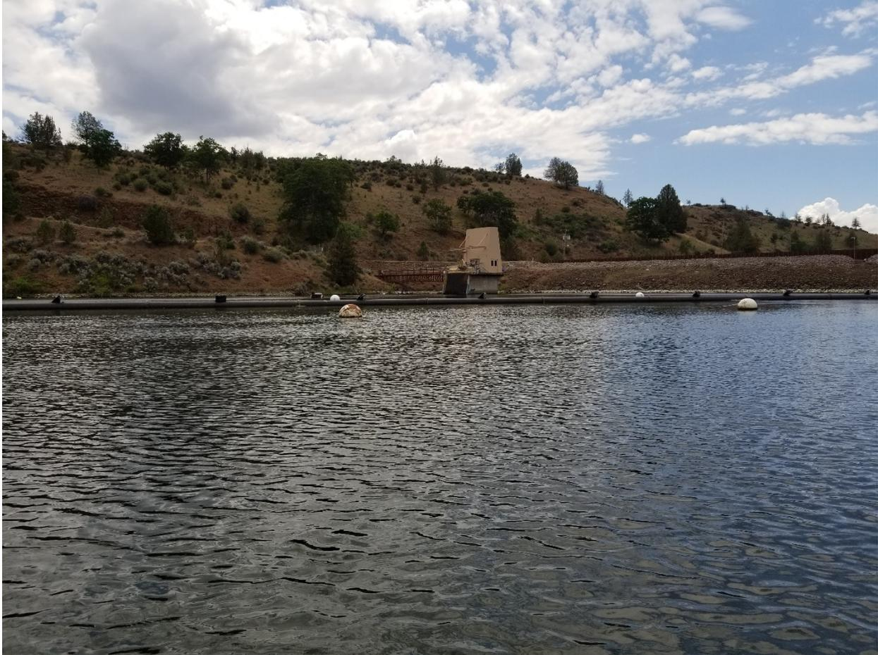
**Figure 2-4. Photograph of barrier curtain surface float (black pipe in center of image), anchor-line floats (white balls on either side of surface float), and intake tower at the southwest corner of Iron Gate Reservoir (taken on May 24, 2018, from the sampling platform upstream of the curtain).**
