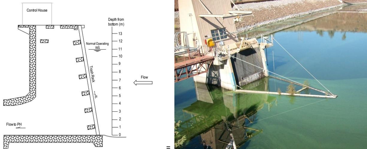
**Figure 2-3. Elevation profile schematic of the Iron Gate Powerhouse intake tower illustrating reservoir operating water surface elevations and vertical extent of trash rack (left) and photograph of intake tower showing open trash rack at reservoir surface (right).**
