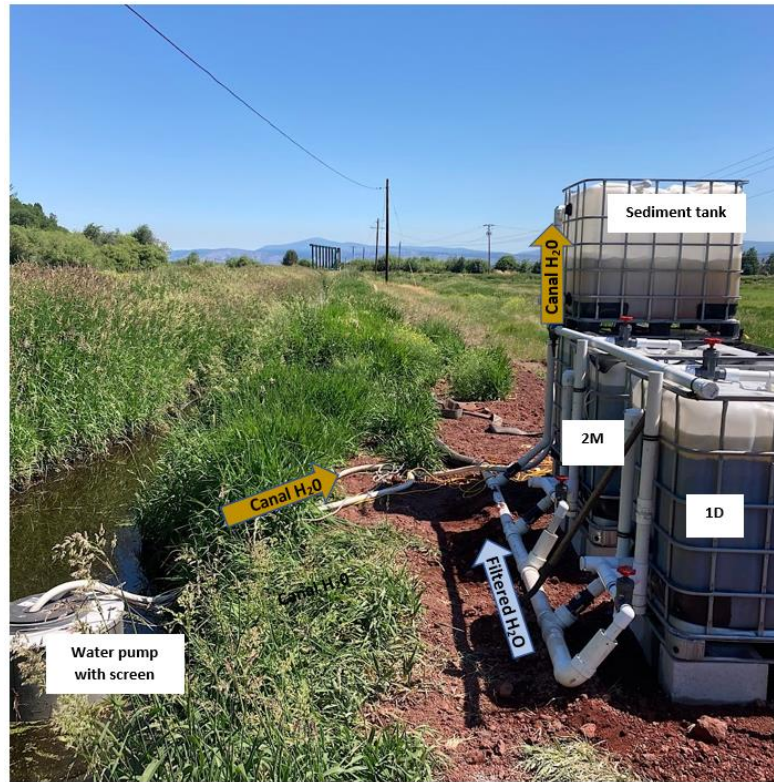
Figure 7. Down flow biochar pilot filter system components (side view)
