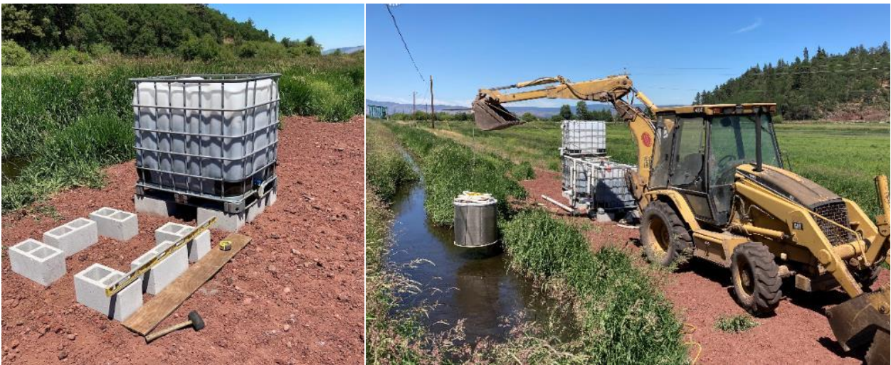
Figure 6. Biochar pilot filter system install
