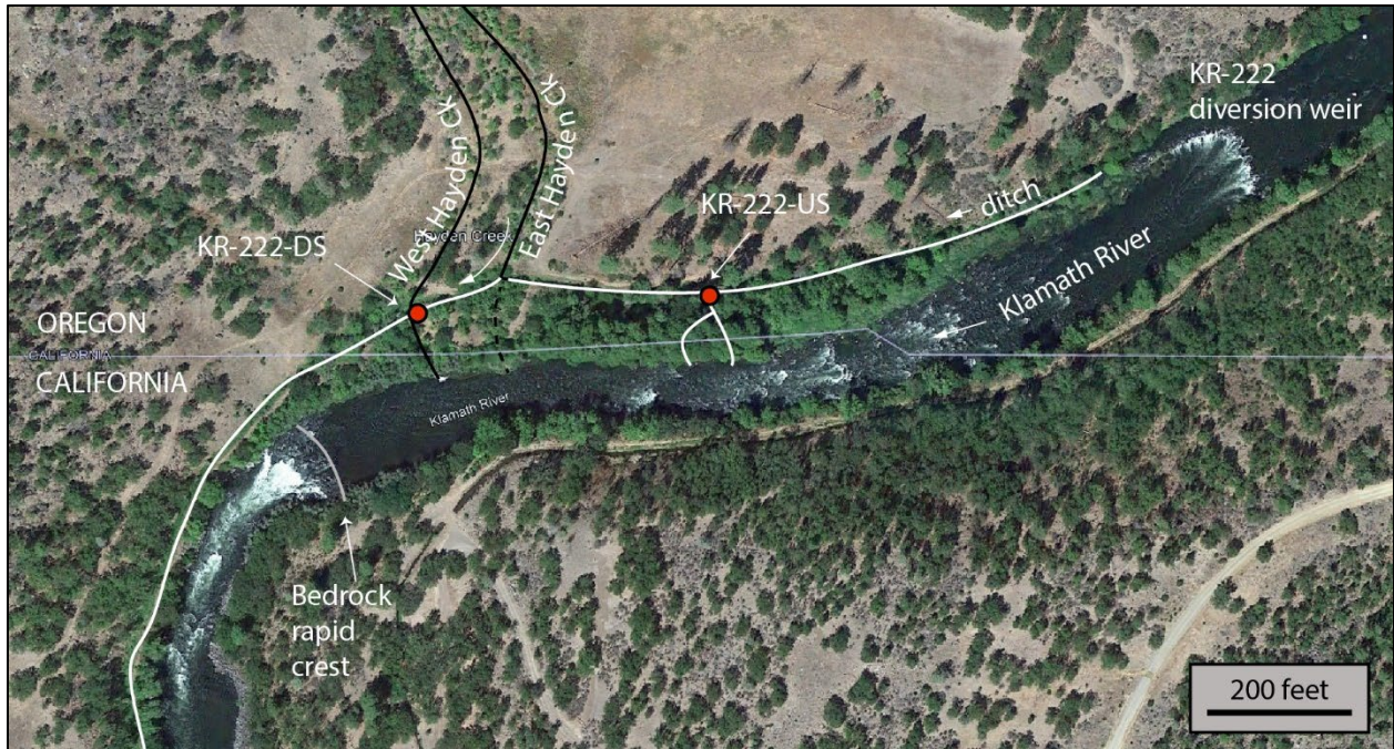
Figure 1-1. Hayden Creek project area. Project area features include ditch and return flow channels (white lines), East and West Hayden Creeks (black lines), historical East Hayden Creek (black dashed line), the bedrock rapid crest (gray line), and the KR-222 controls points (red circles). Feature locations are approximate. Imagery from Google Earth.
