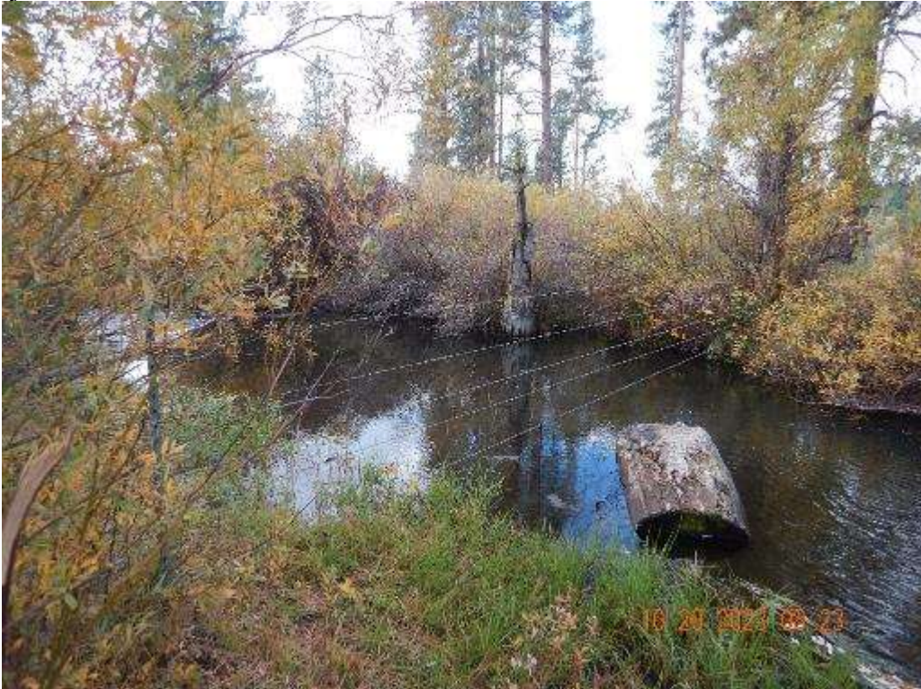
Figure 4. View of the northern intersection of Area 1 fence with Spencer Creek. Fence wires spanning the creek were reattached to T-posts and retensioned.
