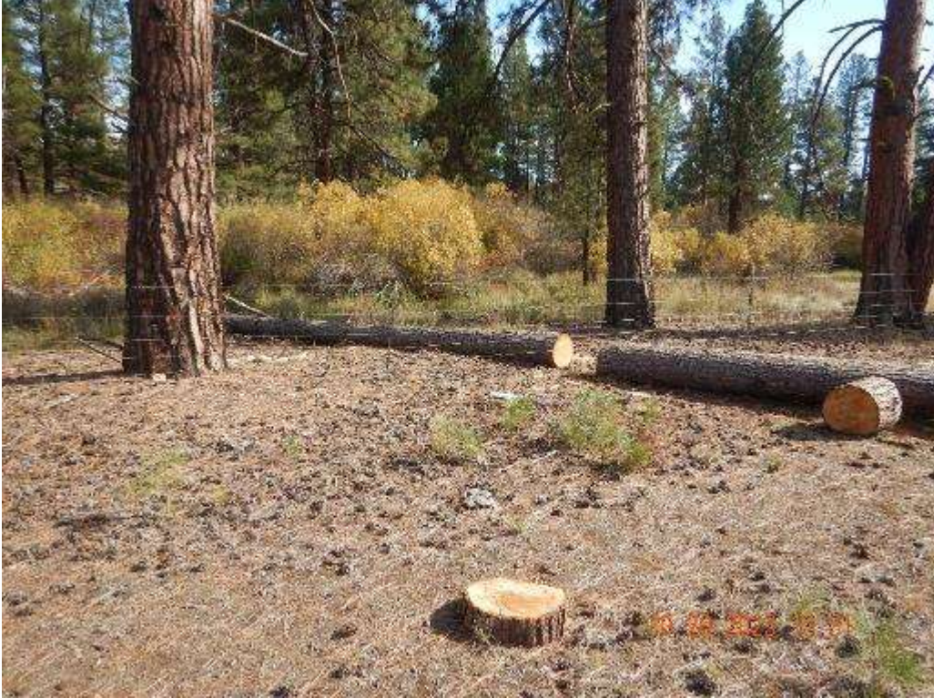
Figure 3. Fallen tree damage in Area 1. A fallen tree was removed from the fence and fence wires were reattached to T-posts and retensioned.
