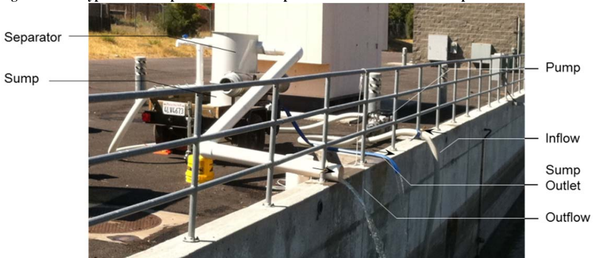
Figure 4. Prototype Particle Separator and its Component Parts – On Site Under Operation
