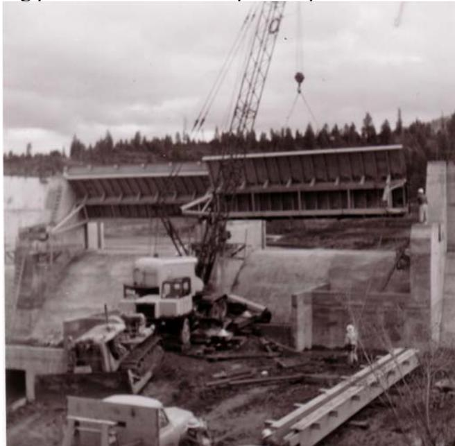
Figure 20: Setting the Tainter Gates
