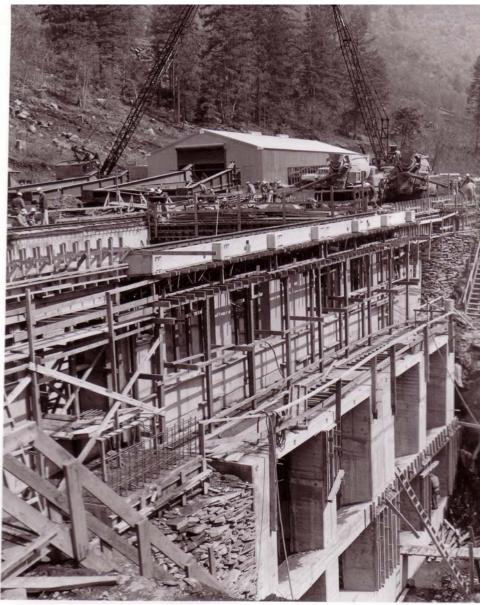
Figure 21: "View of powerhouse where two generating turbines will turn out 80,000kW, April 1958" (Source: PacifiCorp Archive, Big Bend Photographs Vol.5, Neg # BB 695)
