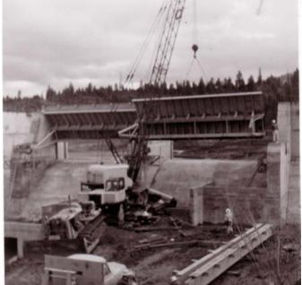
Figure 20: Setting the Tainter Gates Big Bend Diversion Dam, Nov 1956 (Source: PacifiCorp Archive, Big Bend Photographs Vol. 4, Neg # BB 491)
