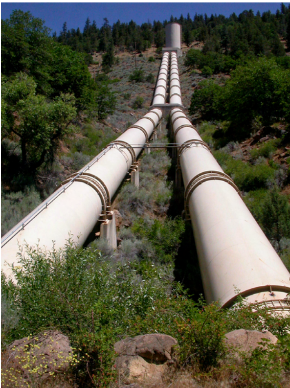
View: J. C. Boyle Water Conveyance System Penstocks and Surge Tank
