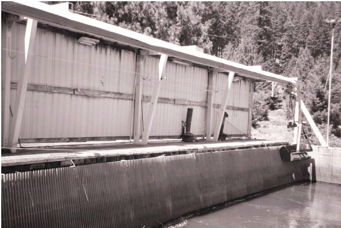
View: J. C. Boyle Waterway Forebay – Floating Spill Gates
