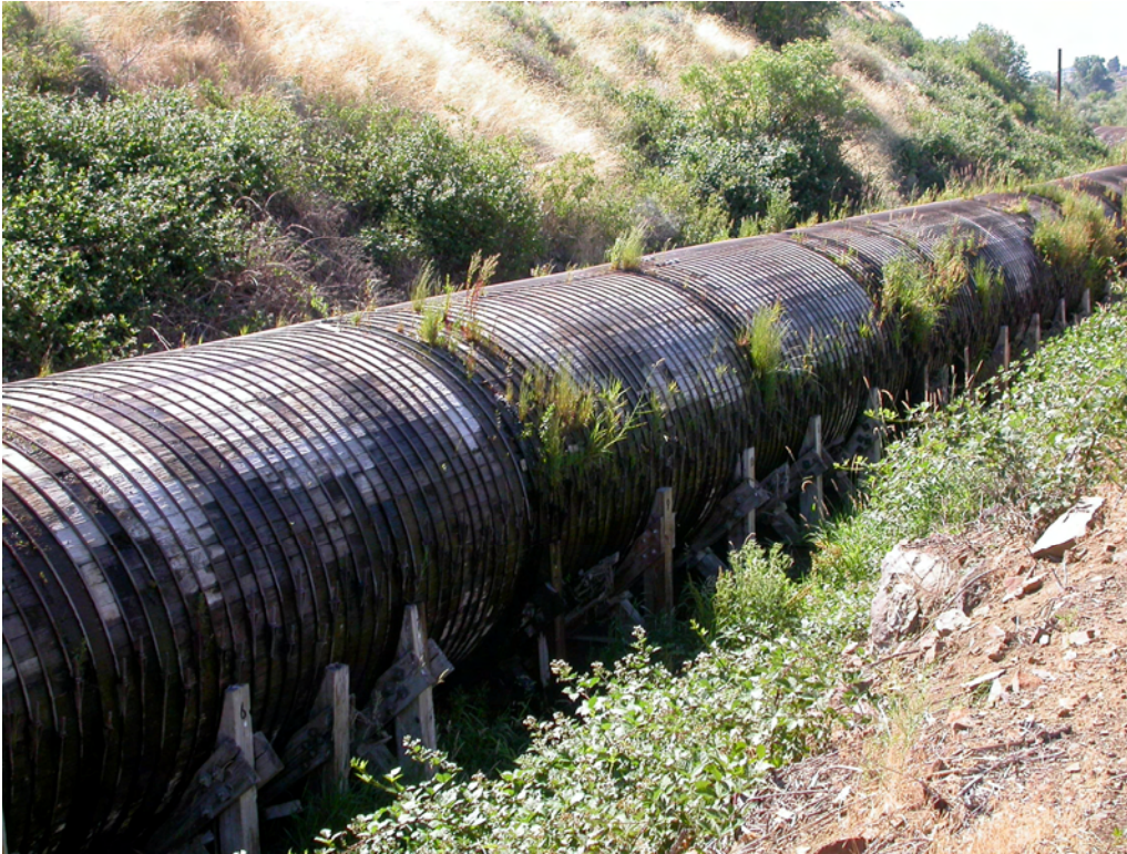
View: Link River Dam East Side Water Conveyance System – Wood Stave
