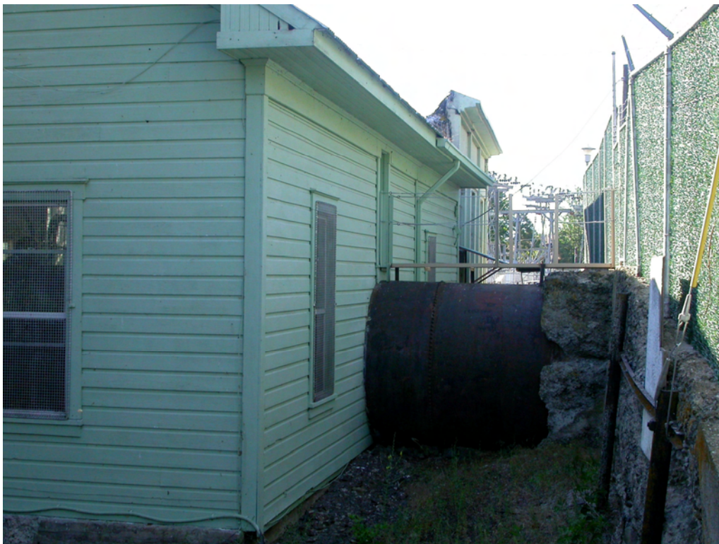
View: Link River Dam West Side Powerhouse, showing penstock entering building
