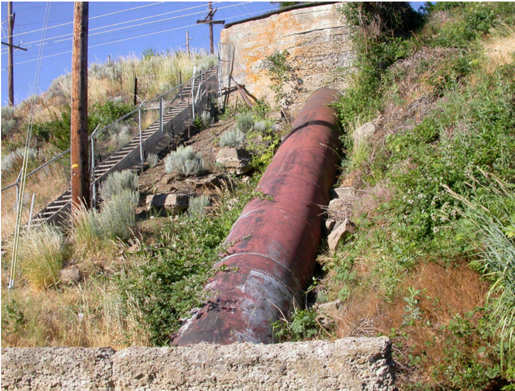
View: Link River Dam West Side Water Conveyance System – Penstock and Concrete Intake Structure
