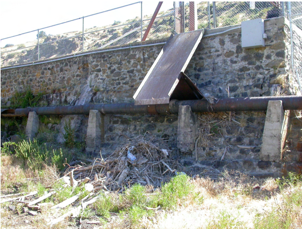
View: Link River Dam East Side Forebay Stone Wall and Trash Chute at Penstock Intake Structure, also showing abandoned fish by-pass on concrete cribs
