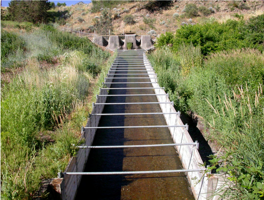
View: Link River Dam West Side Water Conveyance System – Spillway and Concrete-lined Channel to Link River
