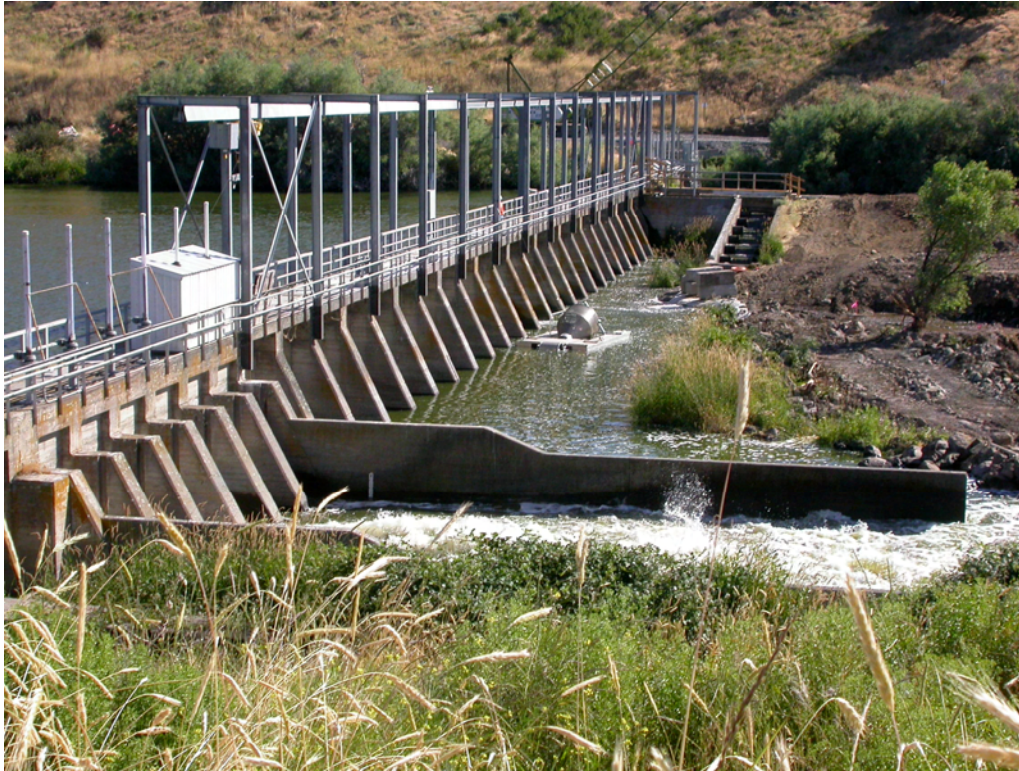
View: Link River Dam from west side, also showing gated West Side Canal Intake Structure
