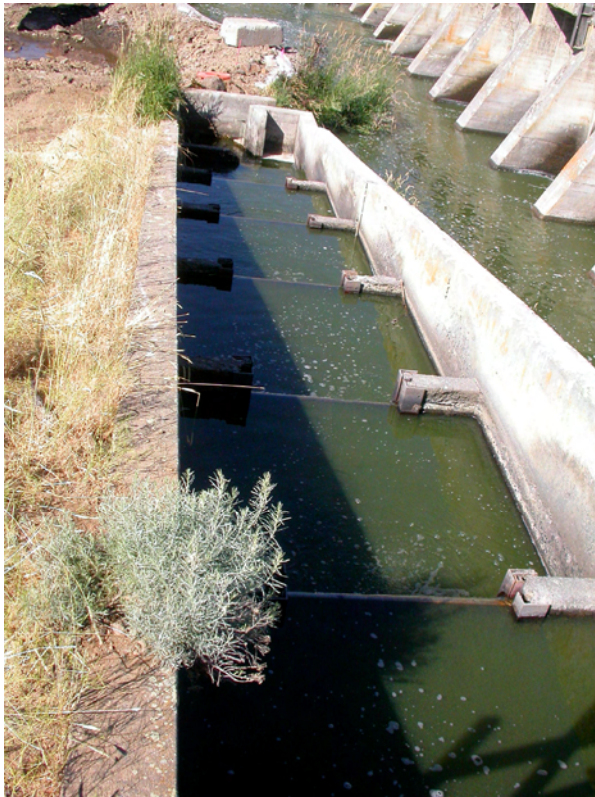
View: Link River Dam Fish Ladder Close-up
