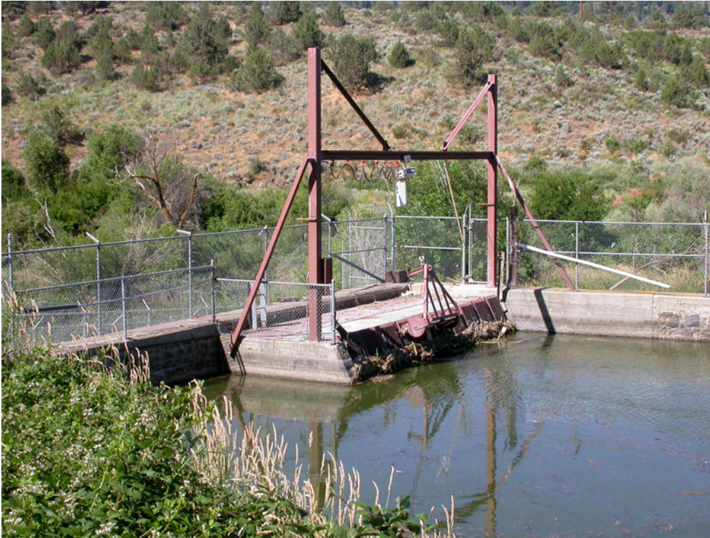
View: Link River Dam East Side Penstock Intake Structure
