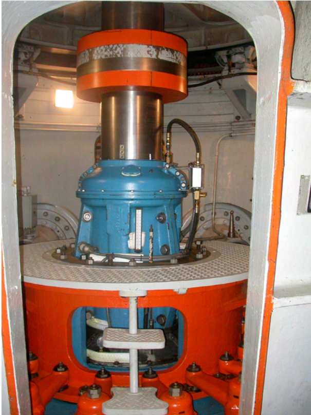
View: COPCO #2 Turbine Unit #1 – in Powerhouse Basement – July 2003
