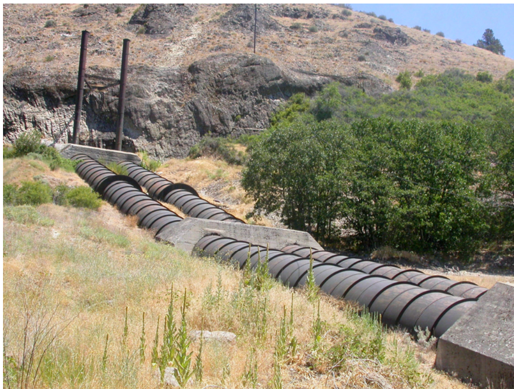
View: COPCO #2 Waterway – Steel Penstocks – July 2003
