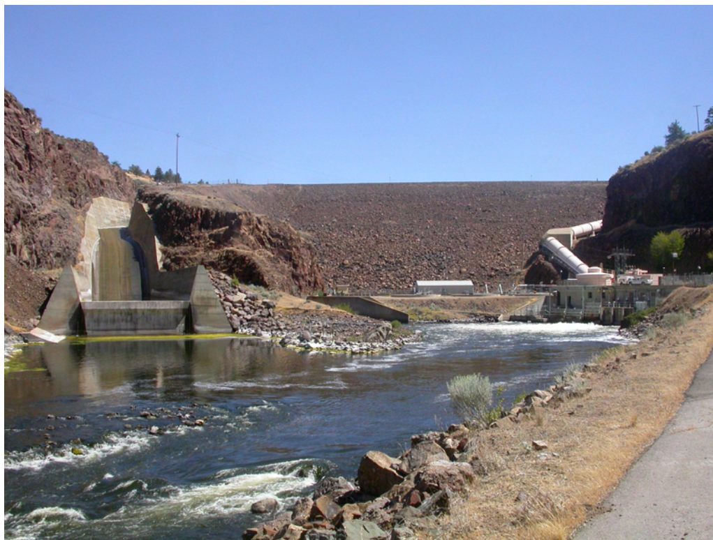
View: Iron Gate Spillway at left - view to penstock at far right - July 2003
