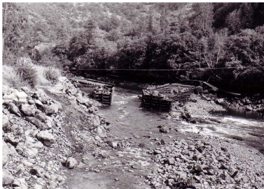
Photo 14. Historic Image COPCO NO. 2 COFFER DAM, c1960 (Source: PacifiCorp Archives )
