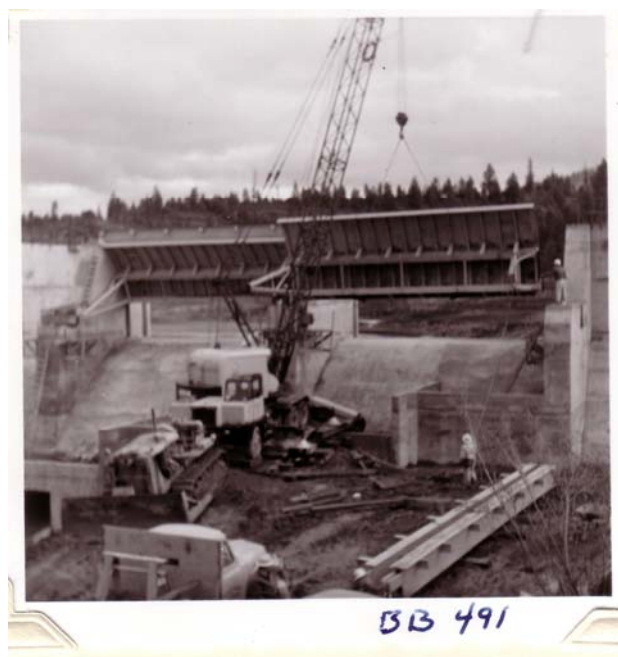
Photo 6. Historic Image BIG BEND (BOYLE) DIVERSION DAM, SETTING THE GATES, c1957 (Source: PacifiCorp Archives )
