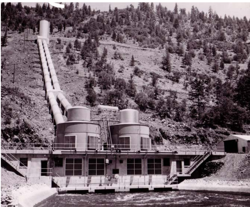
Photo 8. Historic Image BIG BEND (BOYLE) POWERHOUSE, SHORTLY AFTER COMPLETION, C1958 (Source: PacifiCorp Archives )
