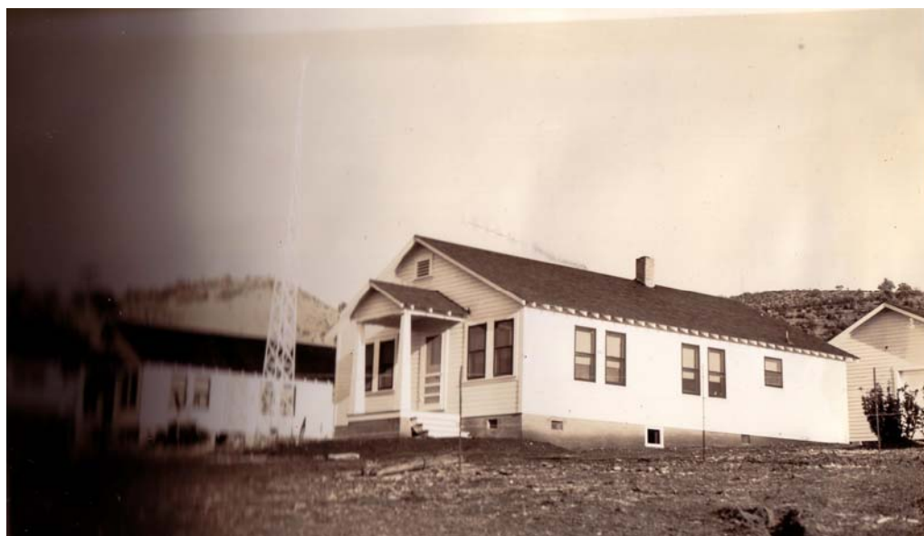
Photo 16. Historic Image COPCO NO. 2 EMPLOYEE HOUSING, c1940 (Source: PacifiCorp Archives )
