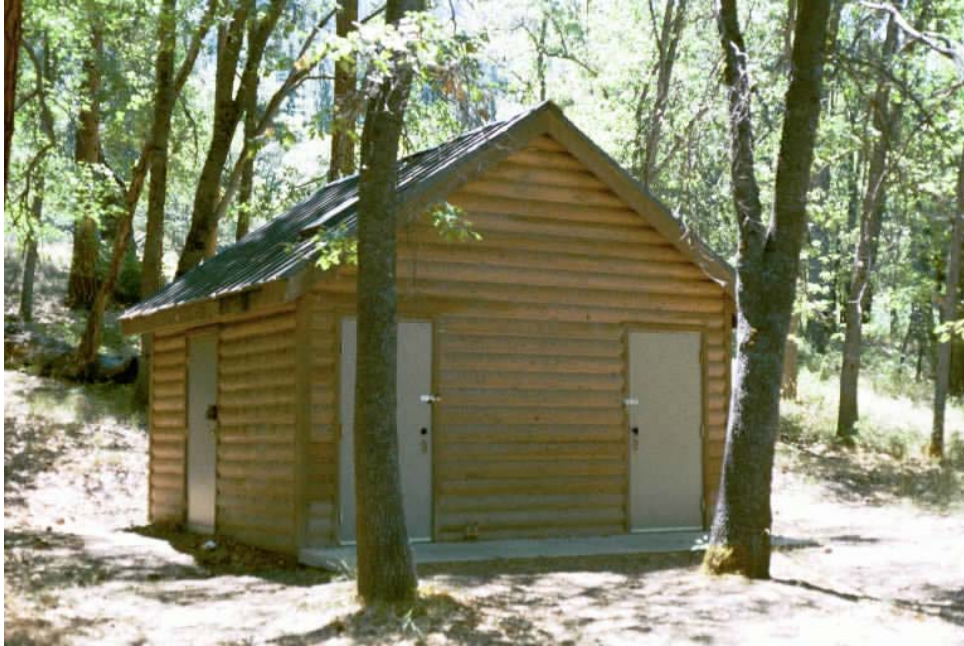
Frain Ranch—Compost Toilet (closed because of vandalism)
