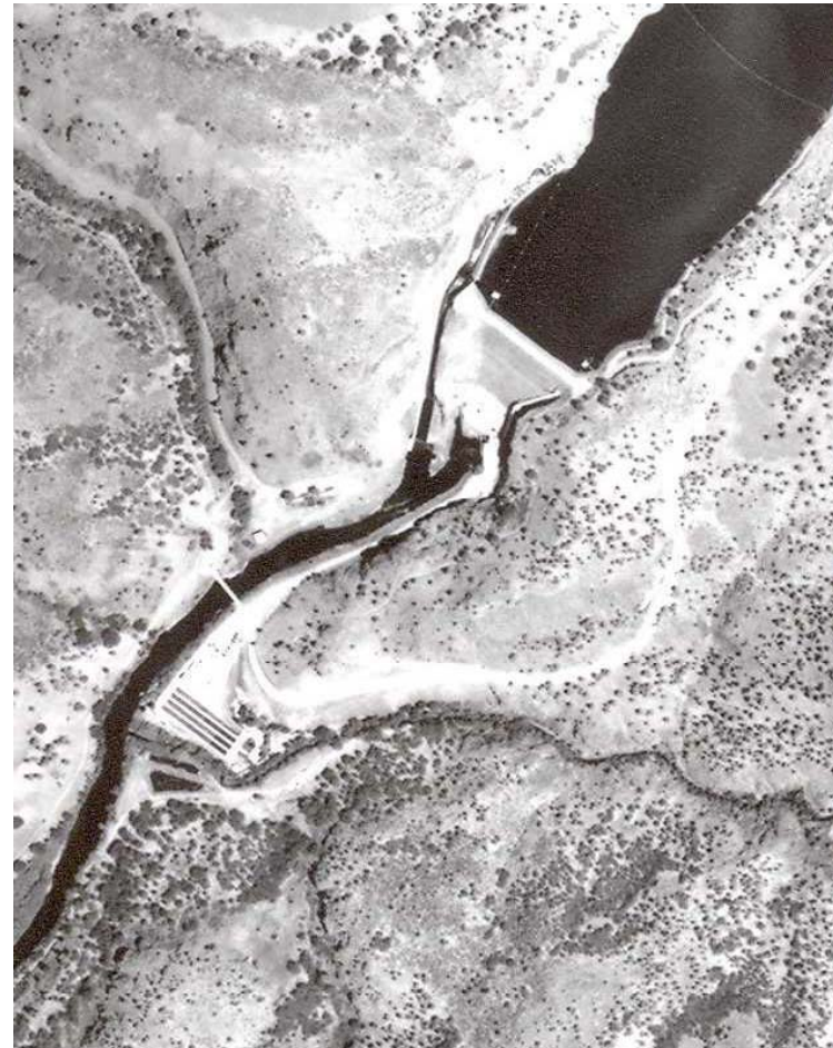
Figure 6.7-35. Downstream of Iron Gate dam (near RM 190) 2001, Q = 1,010 cfs.
