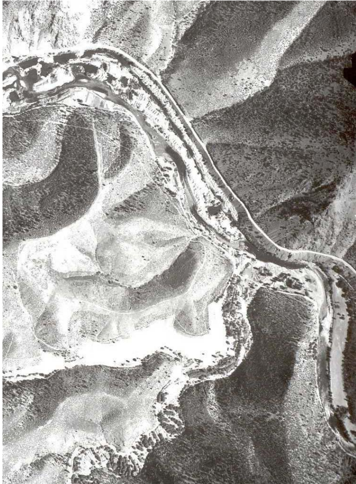
Figure 6.7-38. Downstream of Iron Gate dam (near RM 170) 1955, Q = 1,540 cfs.
