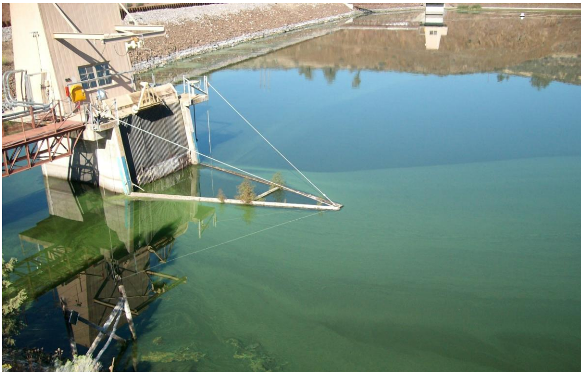
Figure 1. Outlet and trash rack (screen) and surface water entrainment (September 10, 2008).
