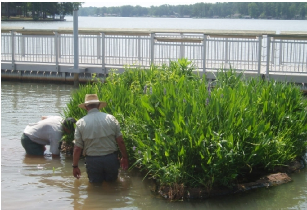
Figure 6. Example of a floating wetland deployment from Lake Sinclair in Georgia (designed and installed by Floating Island International, LLC).
