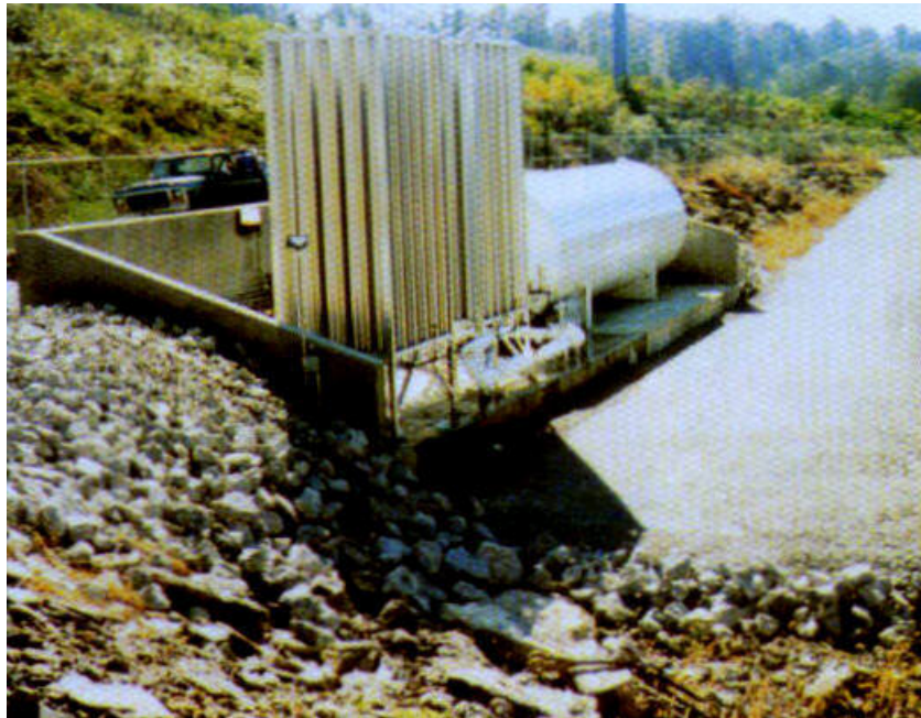
Figure 21: Photograph of a Liquid Oxygen Facility Configured for a Hillside (TVA Tims Ford Dam, 1995)
