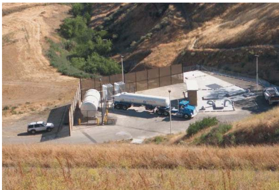
Figure 15: Typical Liquid Oxygen Storage and Supply Facility (Los Vaqueros Reservoir, East Bay Municipal Utility District, Livermore, CA)
