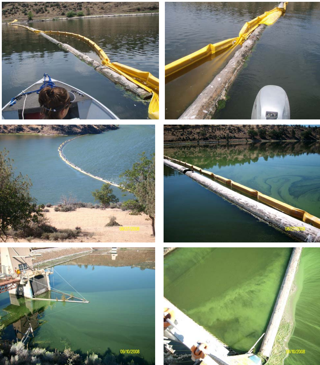
Figure 28. Photographs of the algal barrier curtain in Iron Gate reservoir taken in 2008 (a, b – top row; c, d – middle row; e, f – bottom row).
