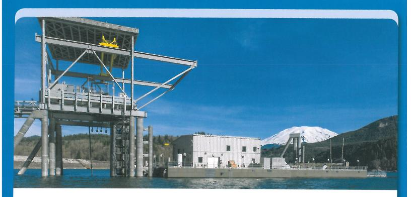
The Swift Reservoir fish collector, located on the uppermost reservoir of PacifiCorp's Lewis River Hydroelectric Project, allows fish moving downstream to make their way to the ocean safely. The goal is to re-ignite migratory fish runs above the three Lewis River dams.
