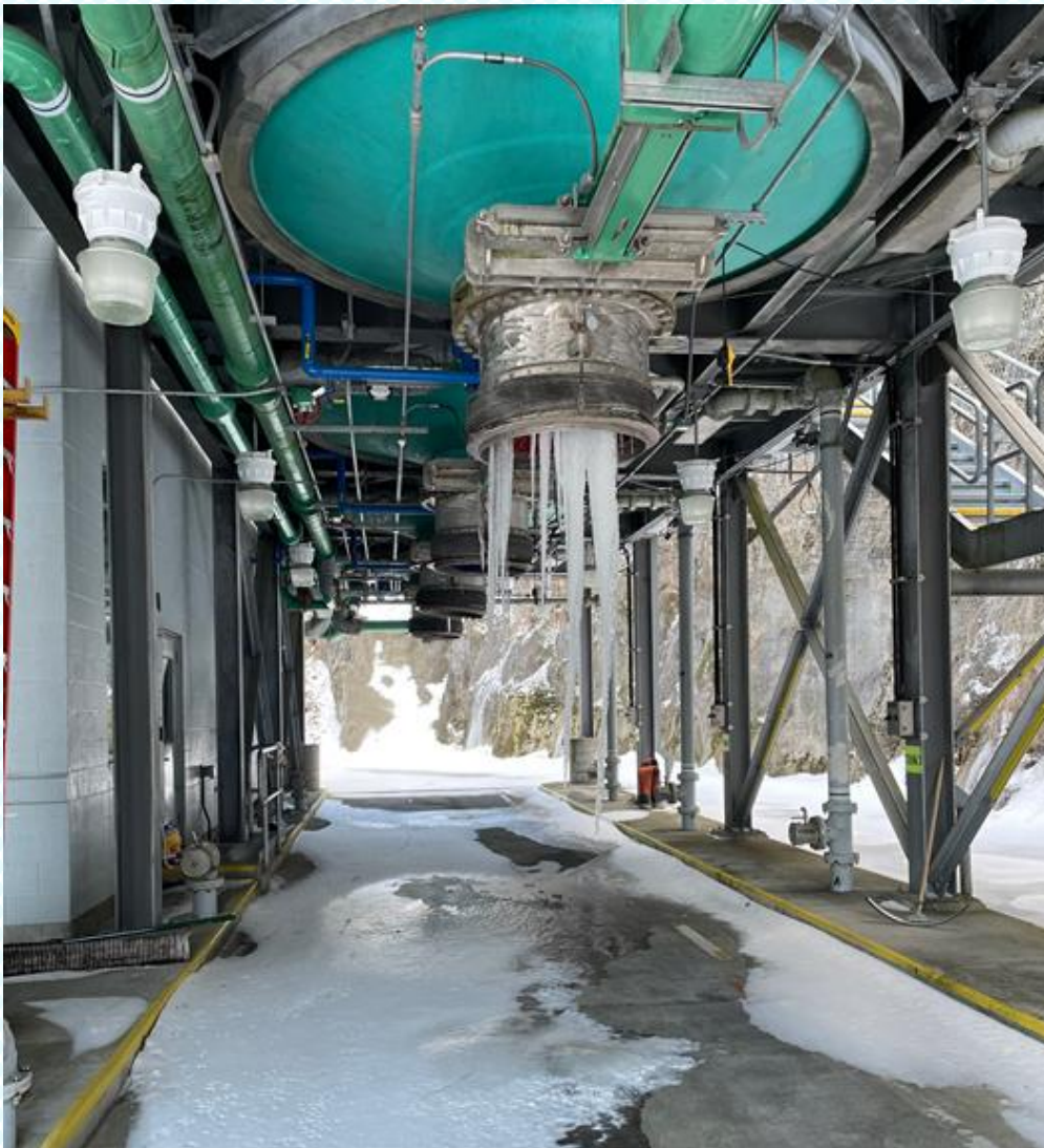
Figure 1. Large icicles hang from a transfer tank at the Merwin Upstream Collection and Transport Facility in January 2024.
