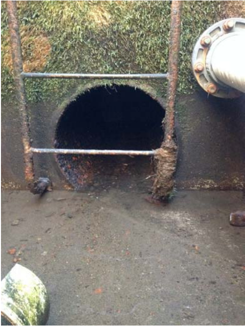
Figure 2: Discharge drain from gallery
