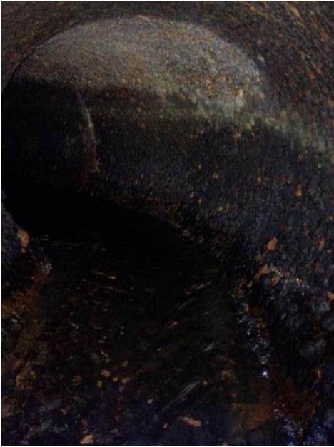
Figure 4: Weir box inlet pipe condition
