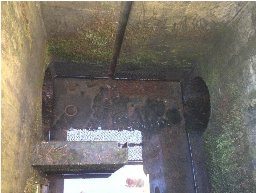
Figure 3: Weir Box indicating incoming pipe from gallery and discharge pipe to river
