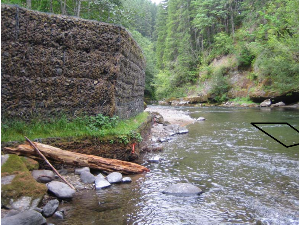
Photo 6. August 19, 2010: Looking Downstream from Bridge
