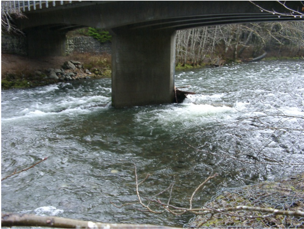
Photo 4. February 7, 2011: Bridge Pier and River Riffle Under Bridge
