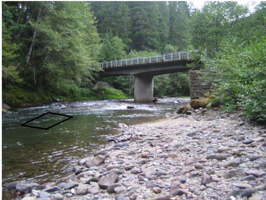
Photo 5. August 19, 2010: Bridge Pier and River Riffle Under Bridge
