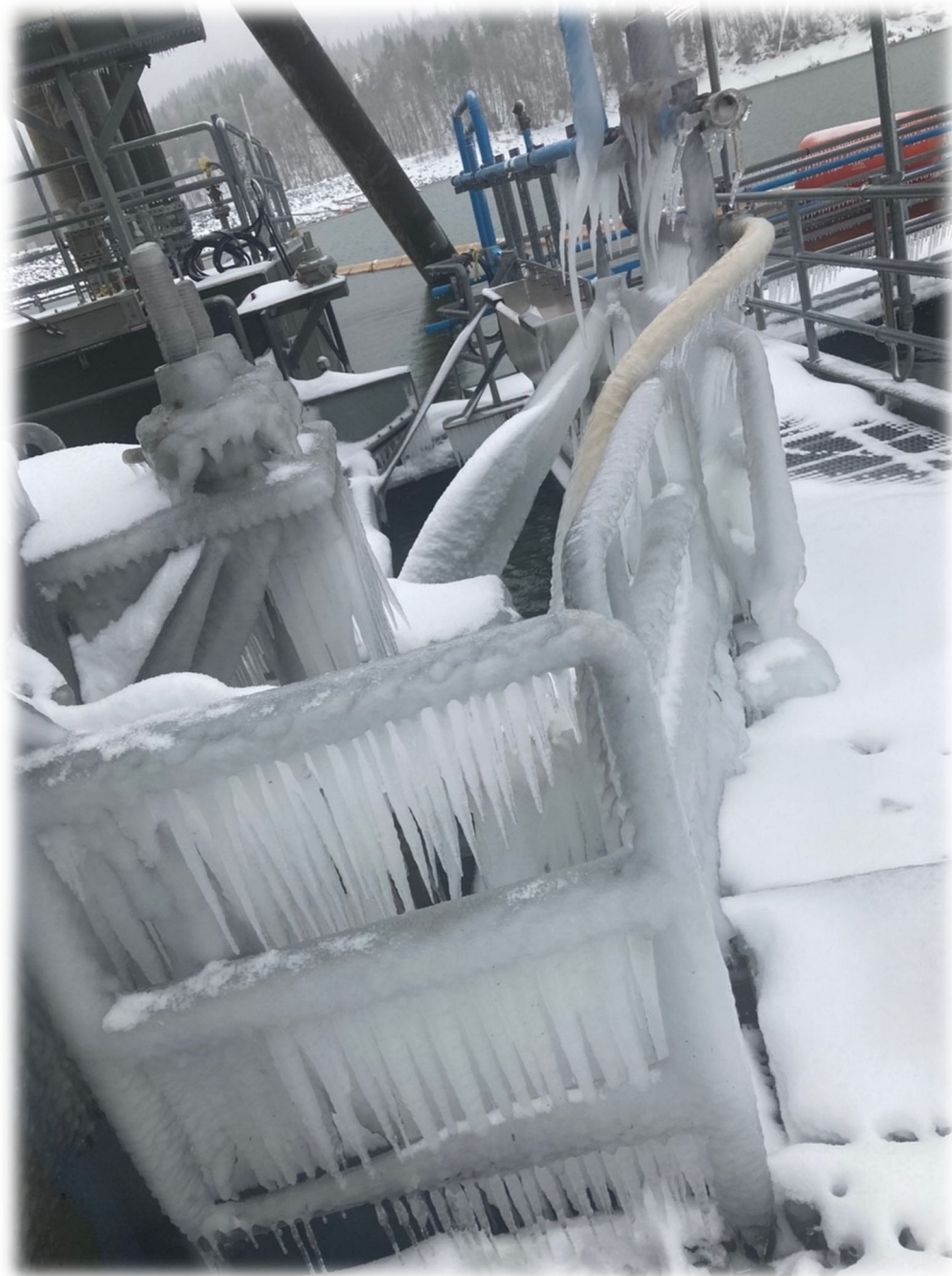
Figure 3. Ice buildup on the Net Transition Structure (NTS) at the Swift FSC following the February winter storm.
