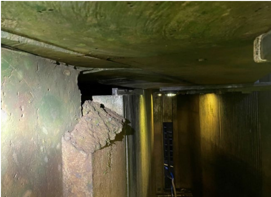
Original image of concrete void as viewed from ladder pool No. 1 - December 22, 2023
