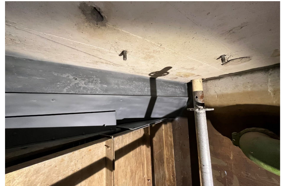
completed plate covering as viewed from the evacuation pump room - March 6, 2024
