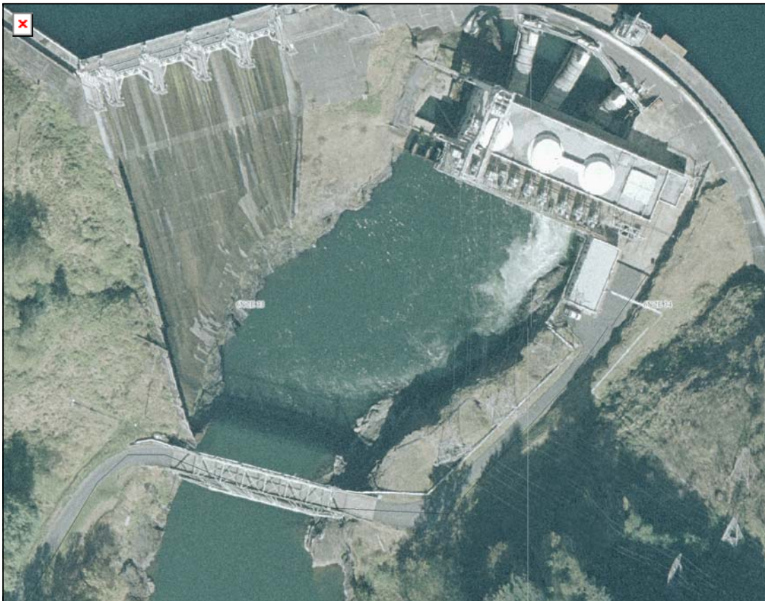
Figure 1. Proposed locations of radio antennas within the Merwin Tailrace.
