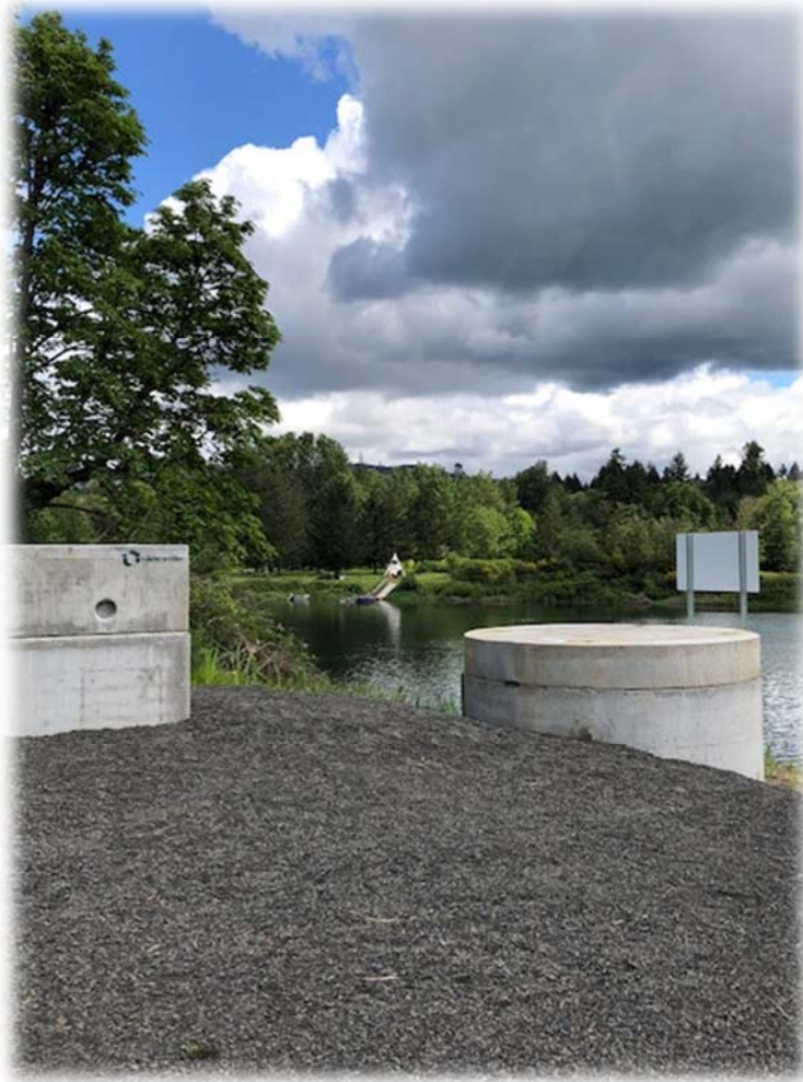
Figure 2. Concrete vaults housing the intake valves and pump inlets for the Lewis River.
