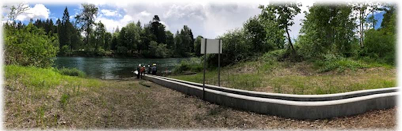
Figure 3. Concrete release flume that transports fish for the raceways to the Lewis River.
