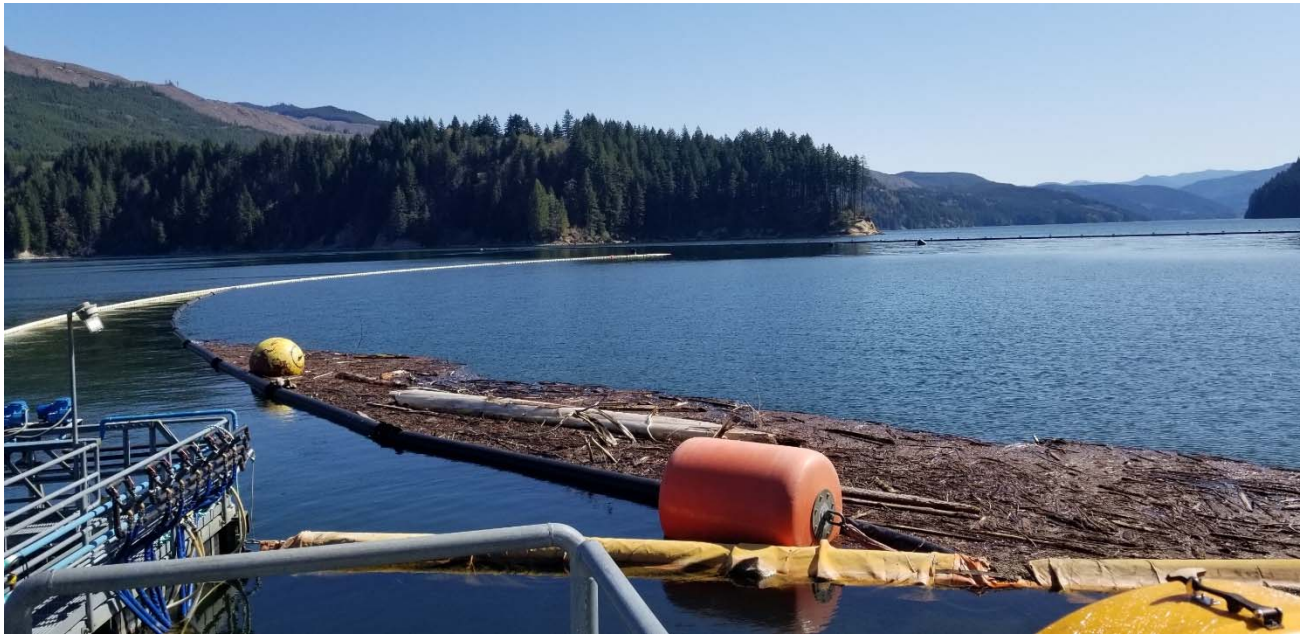
Figure 4. Overnight debris accumulation at the entrance of the Swift Reservoir FSC, May 2020.
