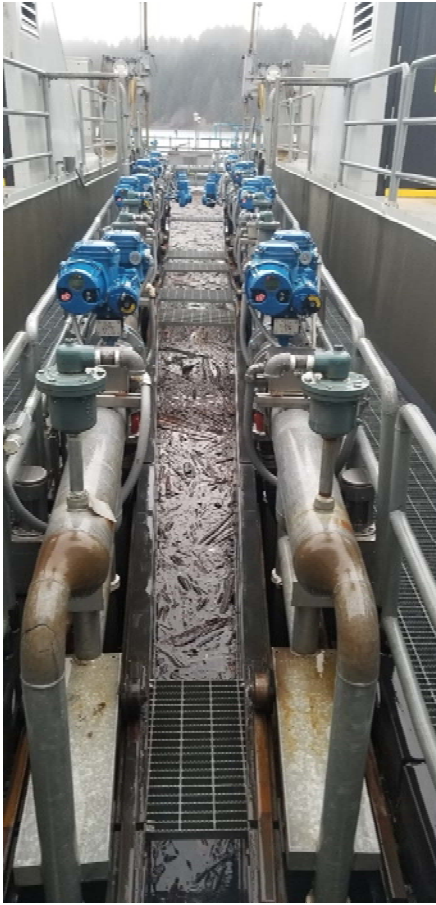
Figure 5. Debris accumulation within the fish passage channel and on separator bars inside the Swift Reservoir FSC, May 2020.
