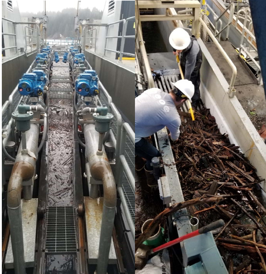
Figure 5. Debris accumulation within the fish passage channel and on separator bars inside the Swift Reservoir FSC, May 2020.
