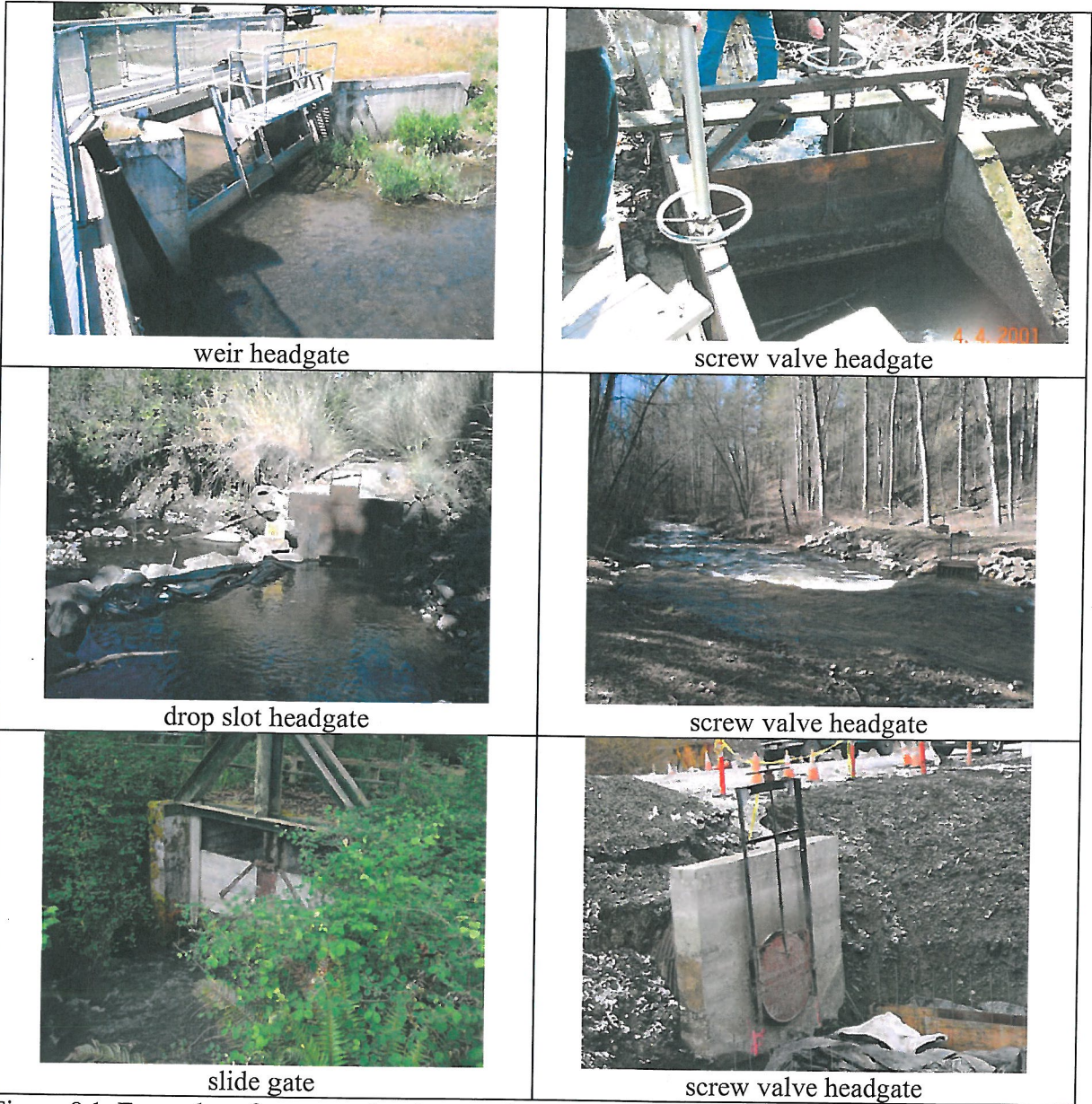
Figure 8.1. Examples of common headgate styles.
