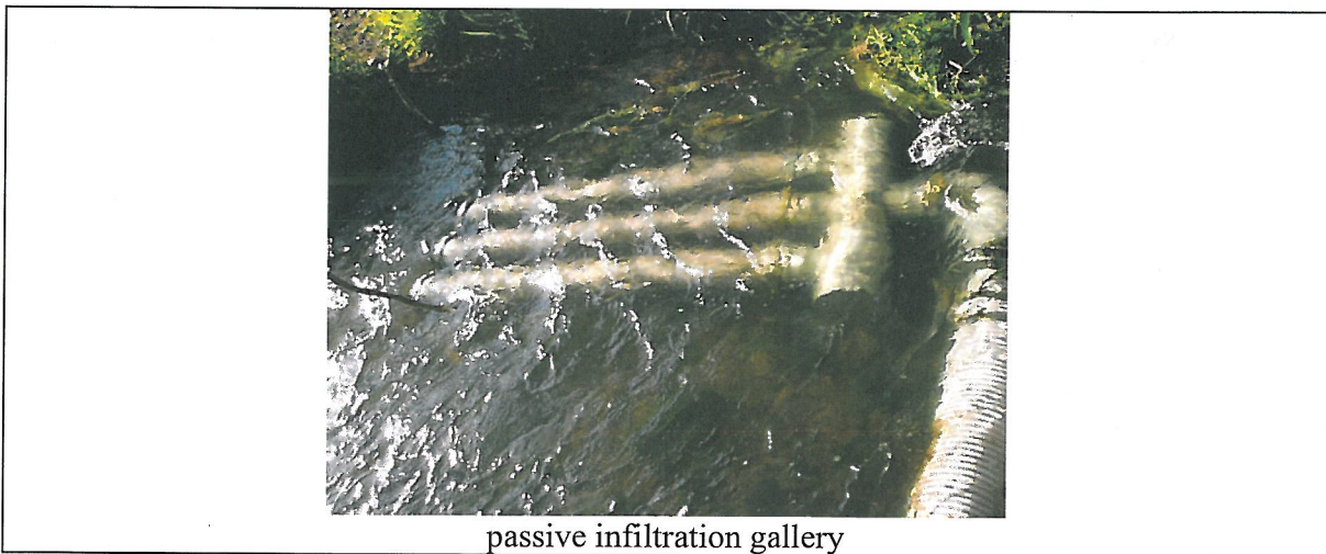
Figure 8.11. Photo example of passive infiltration gallery
