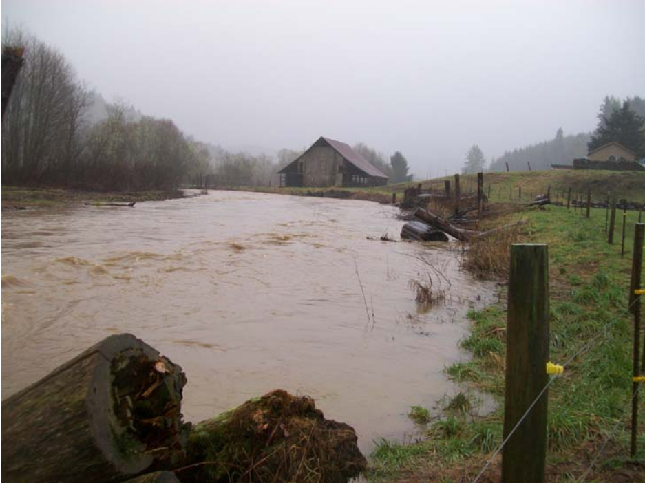
Site during high water event. Jams effectively shift velocity energy off creek bank effectively reducing shear; Project has held up as planned for last 10 years; vegetation fully occupying creek bank.
