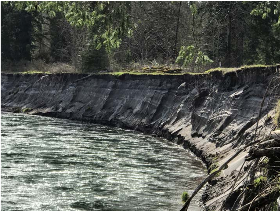
Lewis River bank condition at the proposed project site
