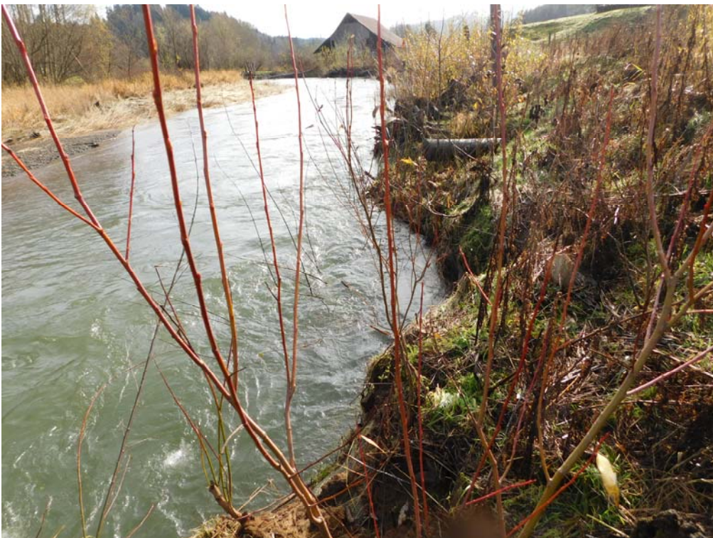
Livestakes after 5-years of establishment; minimum riparian buffer (~25 feet) is providing root strength necessary to hold bank
