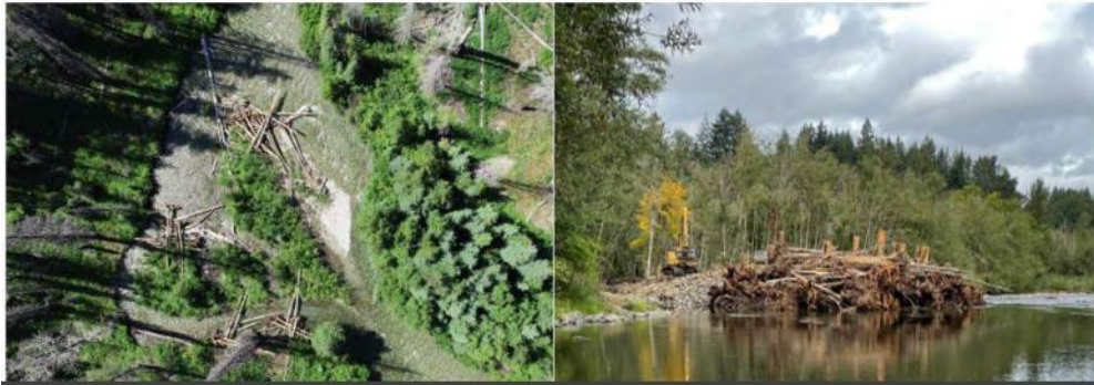
Apex-type wood structures built with a helicopter (left) and ground-based equipment (right).
