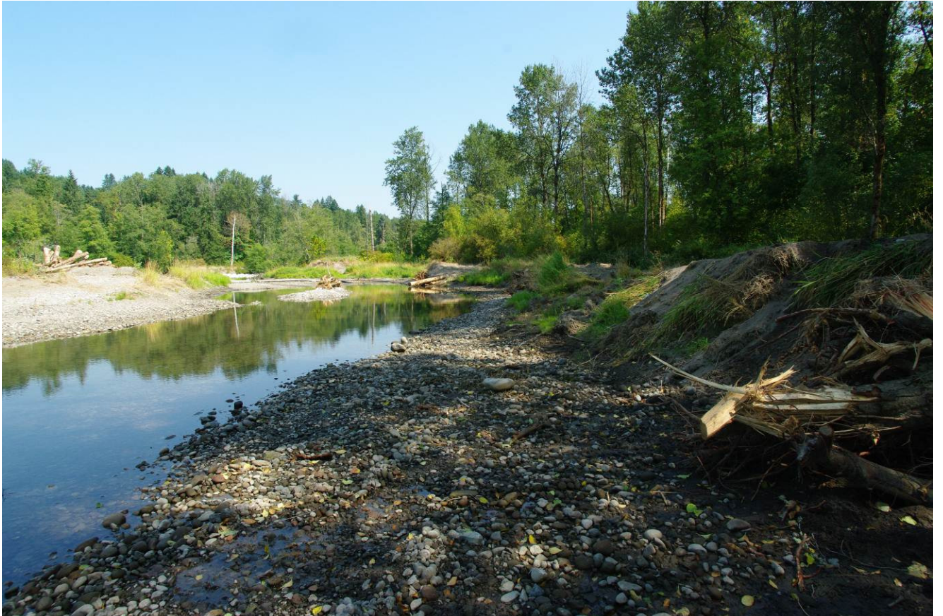
Looking upstream from the south bank of the side channel from the pre-construction photo. Visible on the right are three scour pool structures, in the center a log with rootwad anchored in place, and the head end apex bar jam on the left. Floodplain wood is not yet in place.
