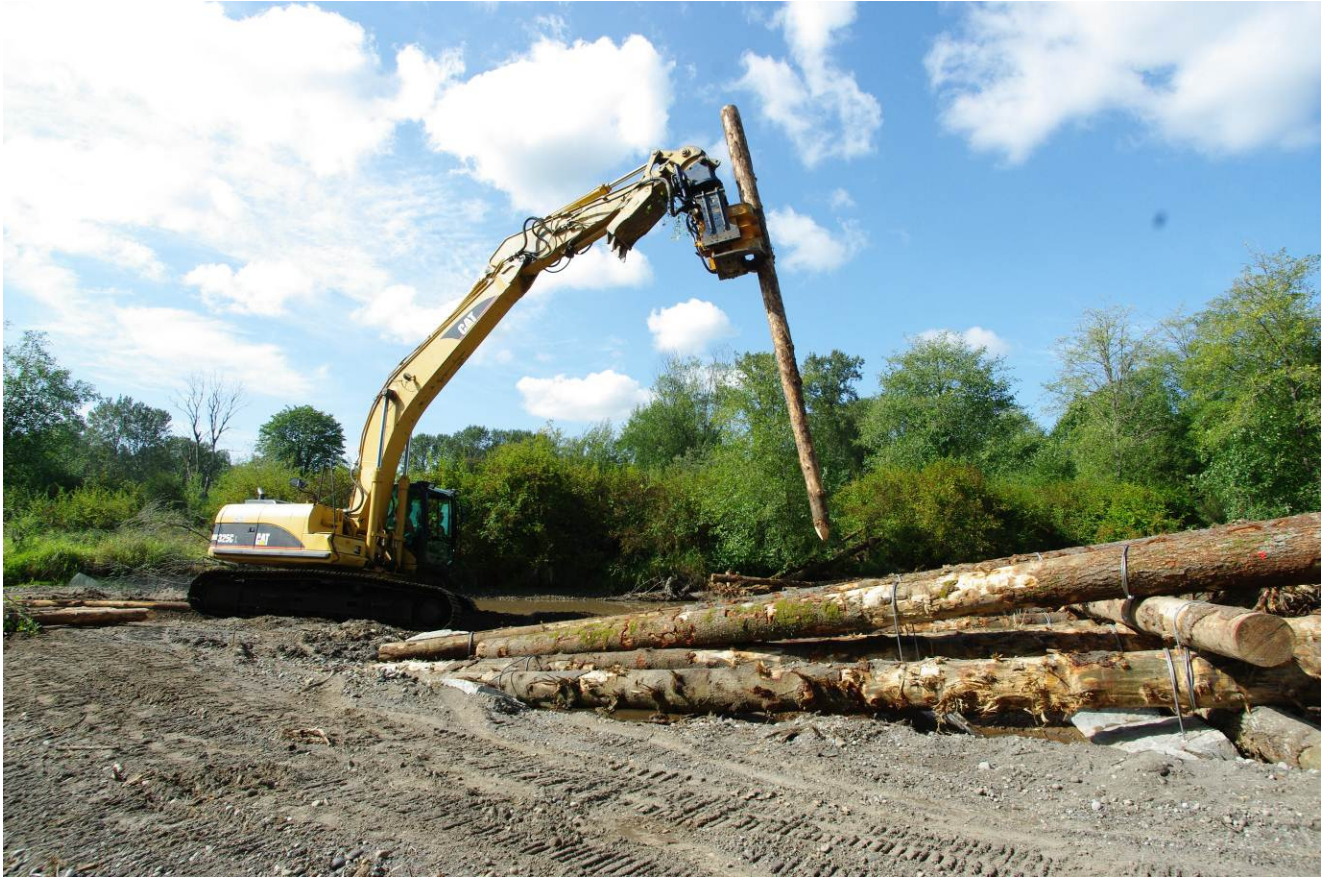
A pile being readied to be driven into apex bar jam #2. This was the typical length and diameter of the logs used as piles
