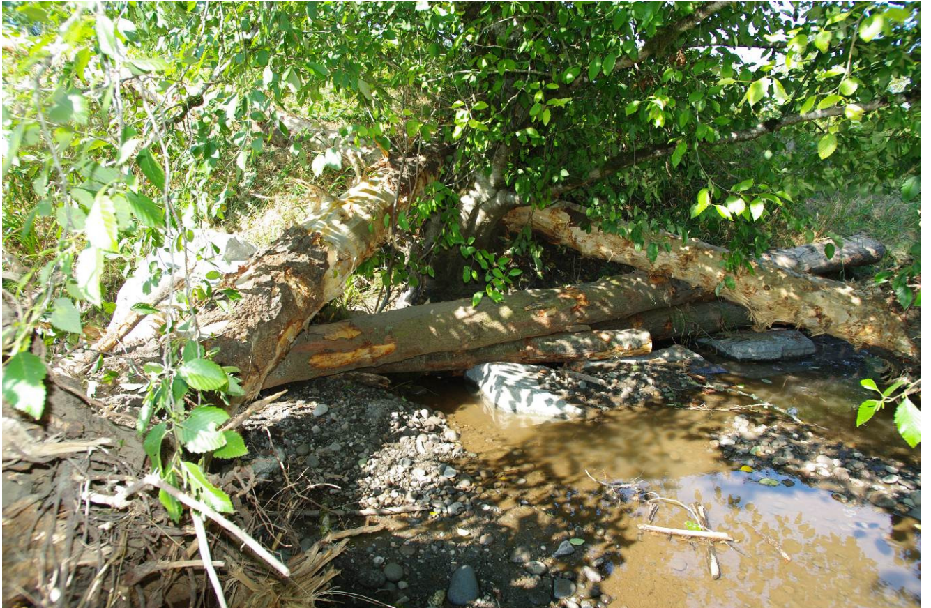
Incorporating an existing alder to make a habitat wood structure
