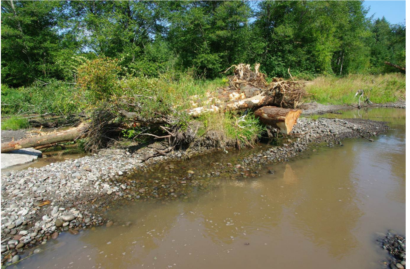
An apex bar jam structure built around an existing alder tree that had fallen
