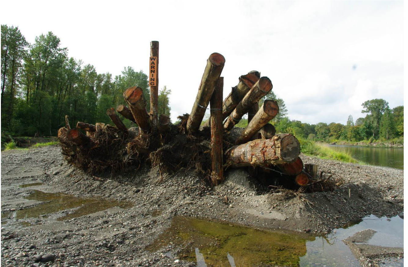
Apex bar jam structure at the head end of the project with warning sign visible. The sign uses 10inch letters and complements the detailed warning sign placed 50 feet out away from the structure.
