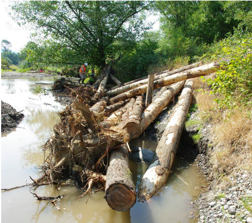
Habitat wood structure being cabled to boulder ballast (not visible in image)
