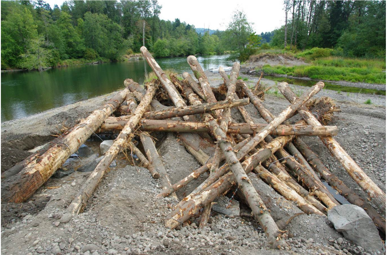
Adding wood pieces to the head end apex jam structure(above), below, looking down at the head end apex jam structure.
