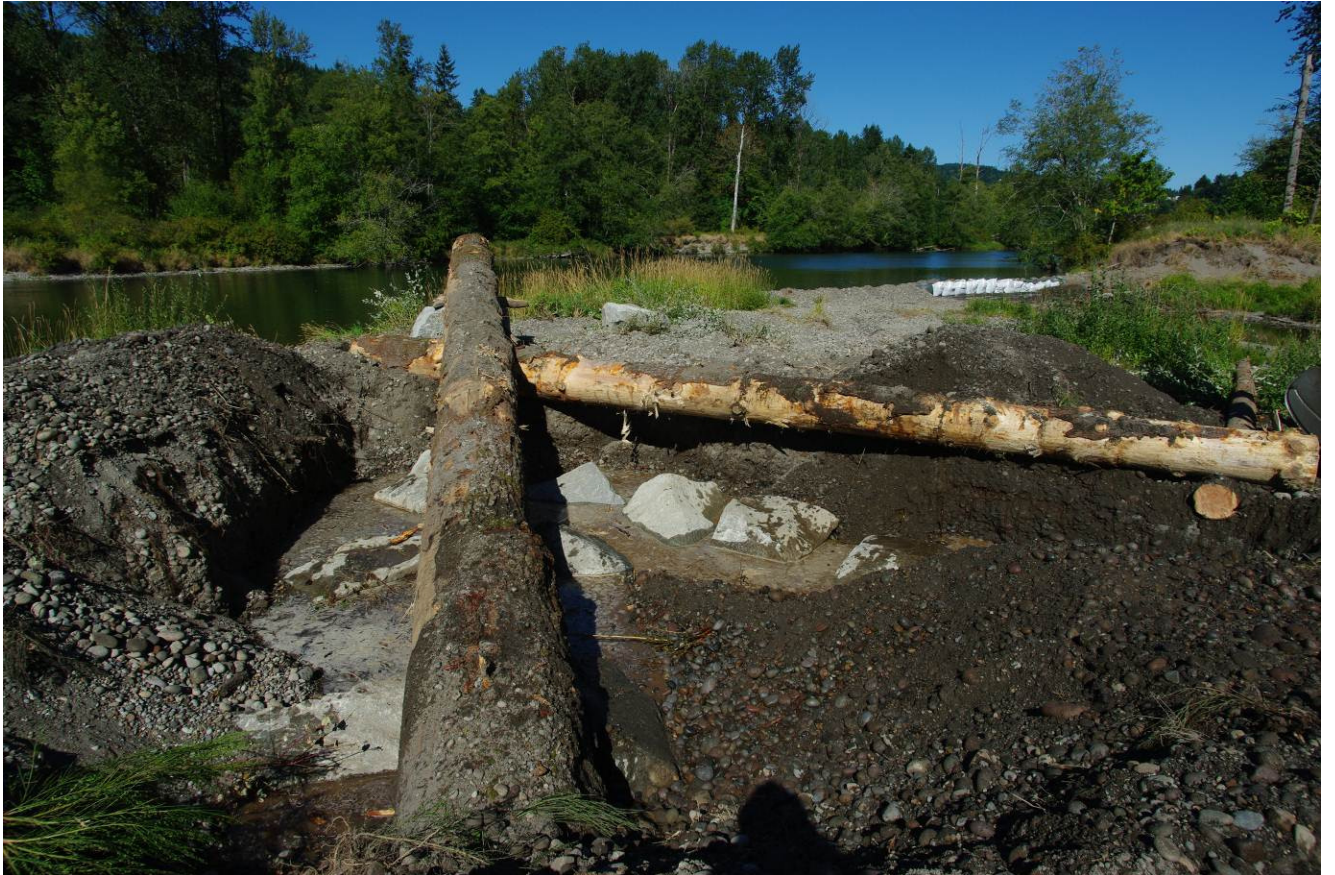
Key log structure of the apex bar jam at the head end of the project. Note the boulders loaded into the excavation in preparation of the next key elements.
