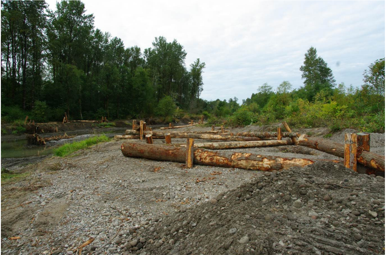
Floodplain wood structures. Consisting of approximately 90 logs, the two floodplain structures (part of the south bank structure is visible here) channel energy into the intended channel at high flows
