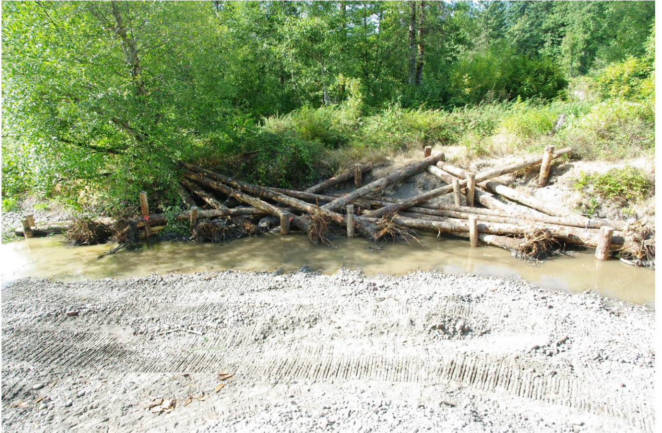
Habitat wood structure
