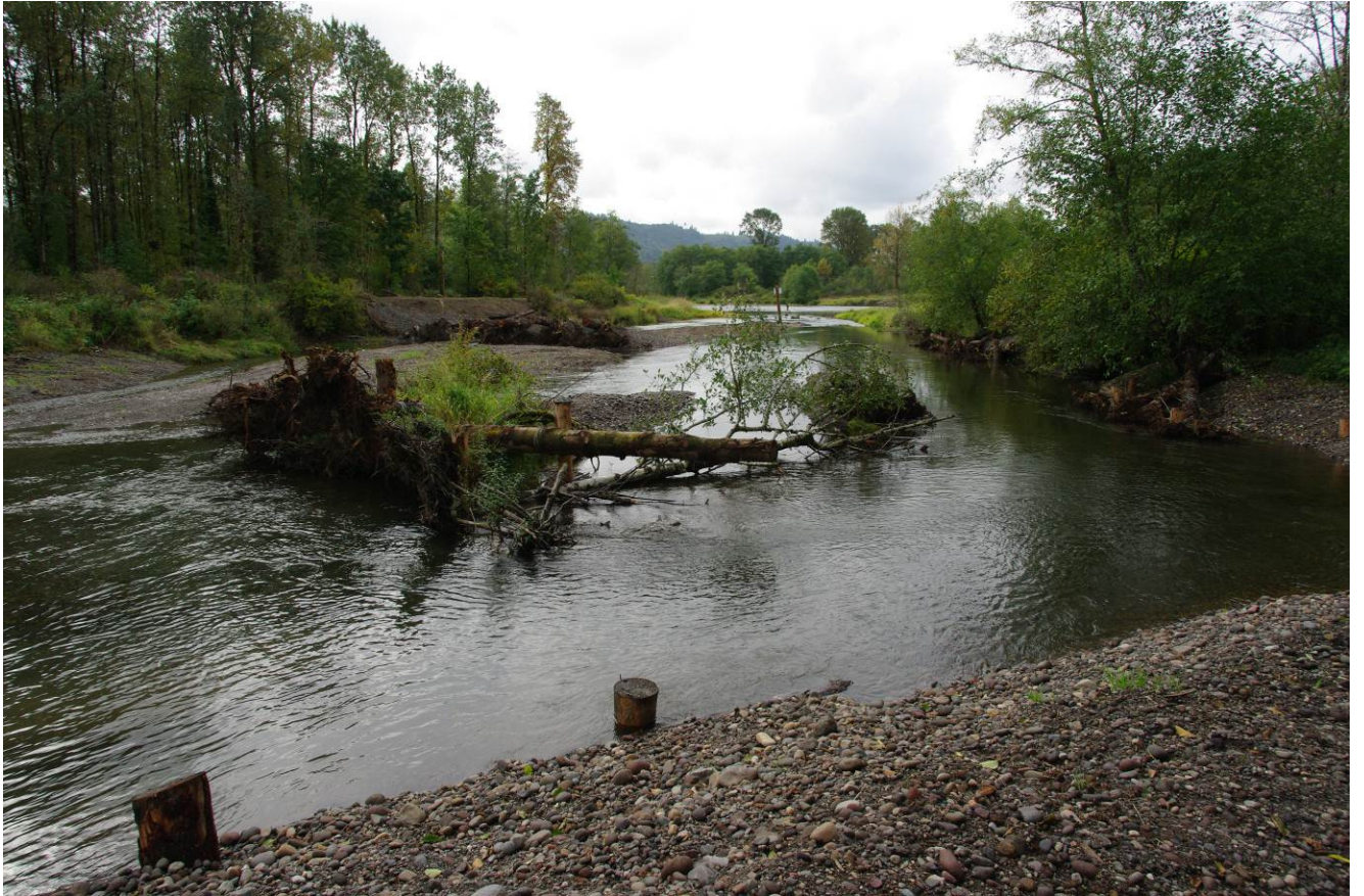
Looking downstream to the tail end of the project from near the center of the project after construction was completed.
