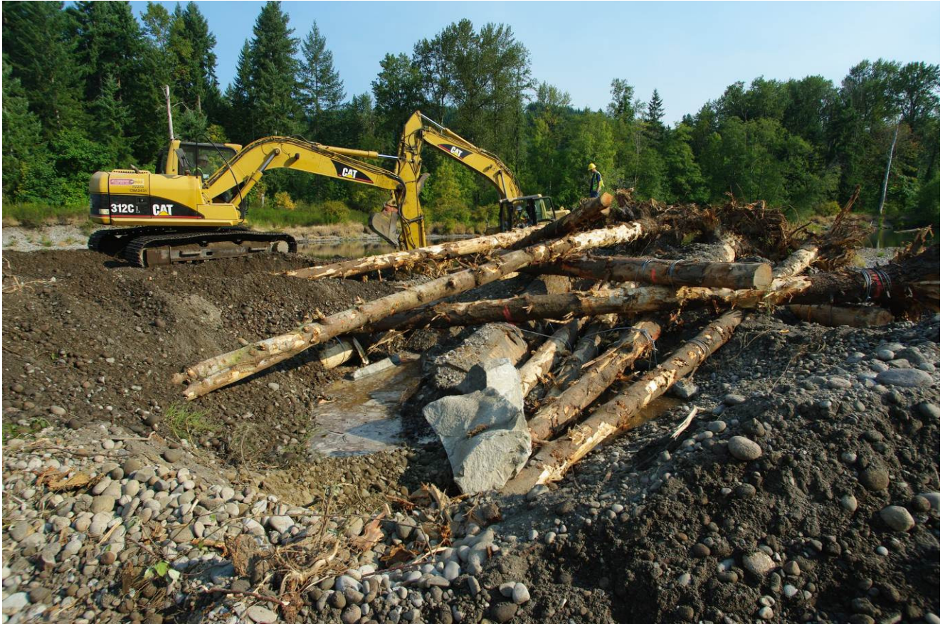
Adding wood pieces to the head end apex jam structure(above), below, looking down at the head end apex jam structure.
