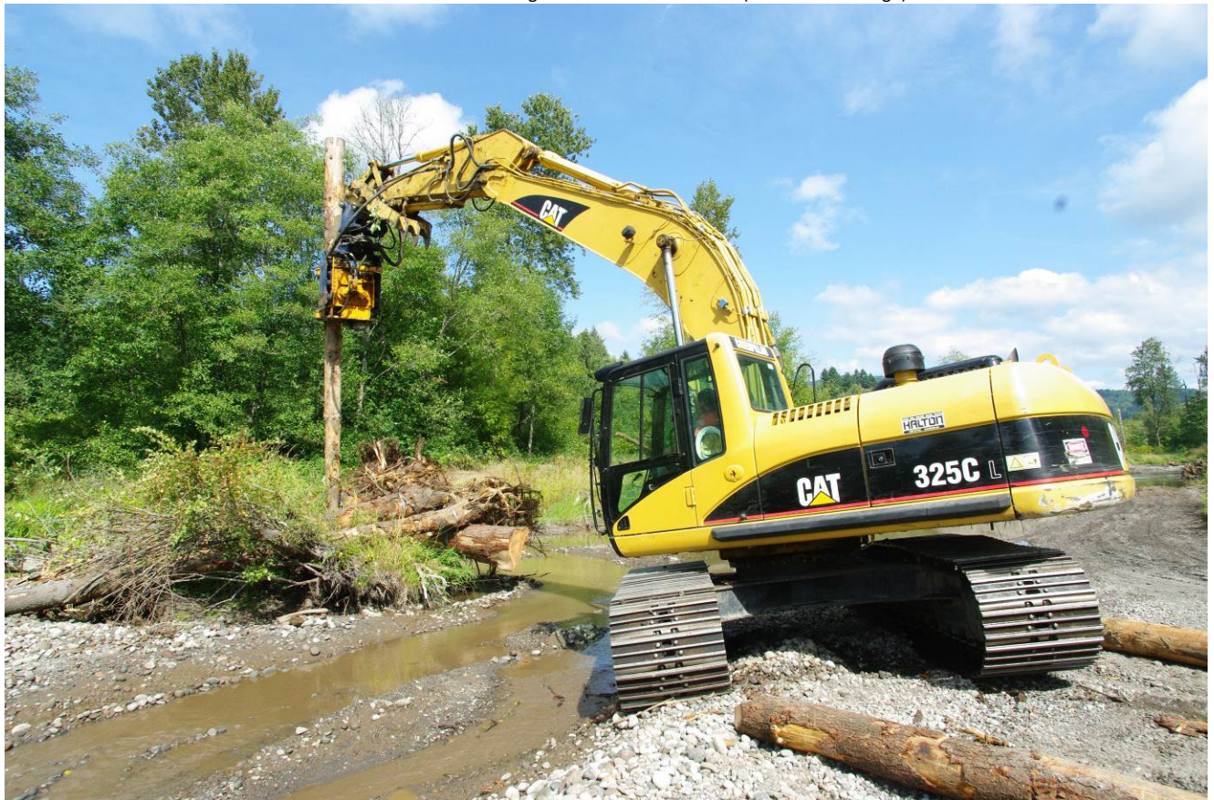
Pile being driven into apex bar jam number three. There were four apex bar jam structures built into the project.
