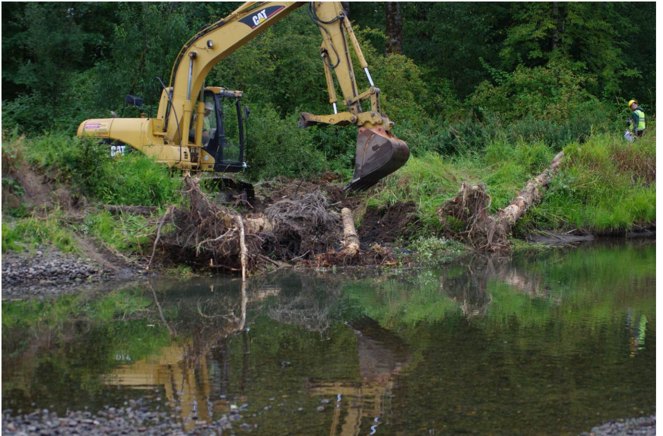
Installation of an upstream scour pool structure. This structure was buried and ballasted into the bank.
