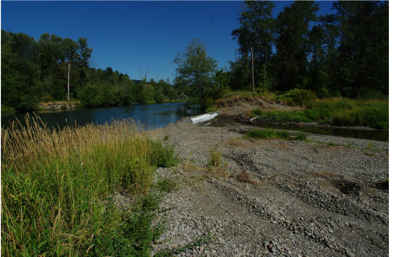
Upstream coffer dam. The entire project site was dewatered and kept from "live" water throughout the entirety of the construction phase.
